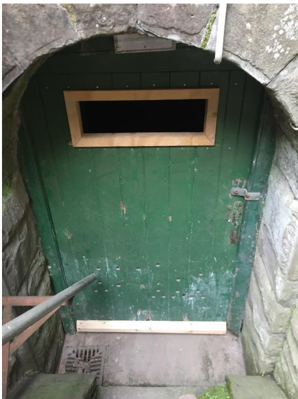
Cellar door following installation of bat access slot spring 2020
