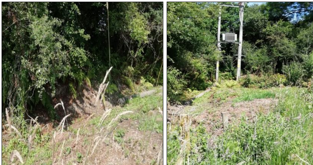
Figure 6. Cleared area around pylon footings, with dry ditch banks
