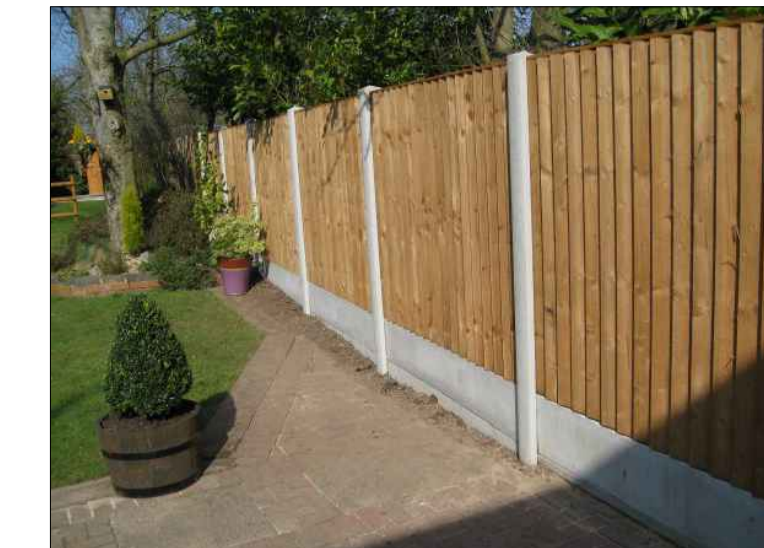
1.8m High Timber Closeboard Fence with Concrete Posts
