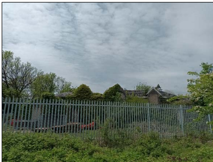
Plate 12 – Building 2 at the northern end of the fenced compound area.
