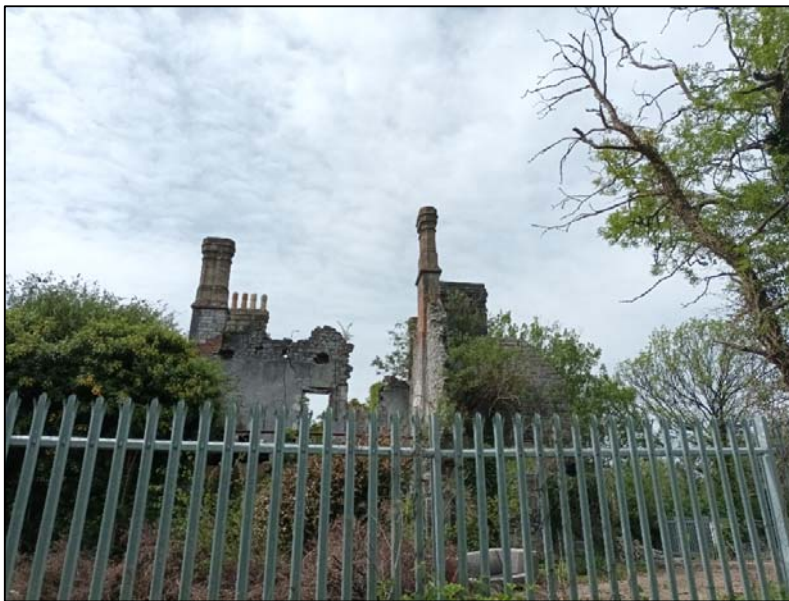
Plate 11 – Building 1 at the southern end of the fenced compound area.
