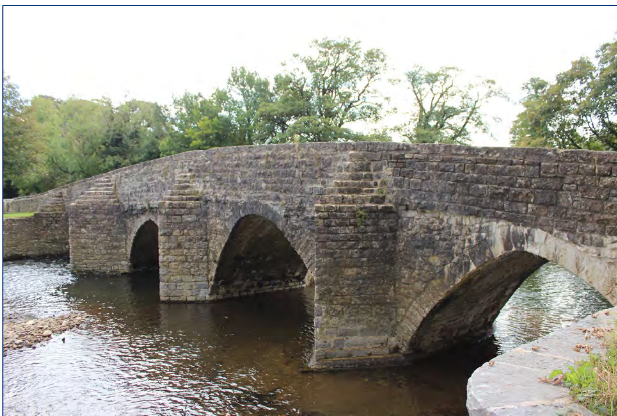
Plate 17: New Inn Bridge looking south.
