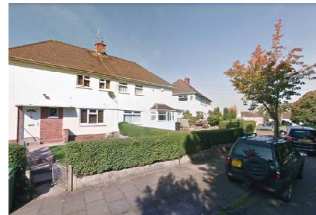
Plas-Mawr Road (immediate context) 2-storey, hipped roof, brick and render.
