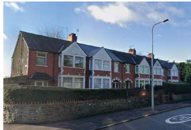
Fairwater Green. Roof with eaves at the front, utilizing small gables to break the rhythm of the facade.
