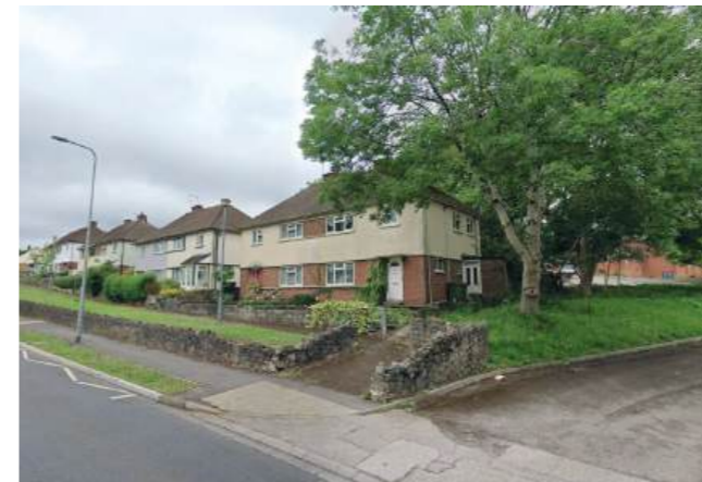
Ferrier Avenue (immediate context). 2-storey, hipped roof, brick and render.
