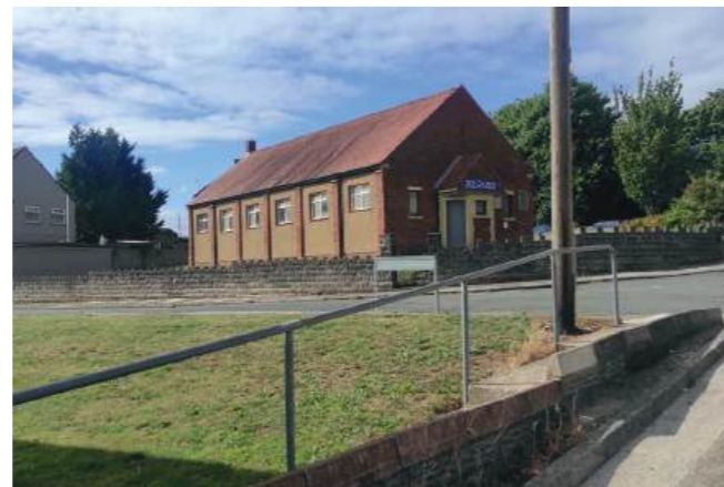
DCF Church (immediate context). Pitched roof, using brick as main material.
