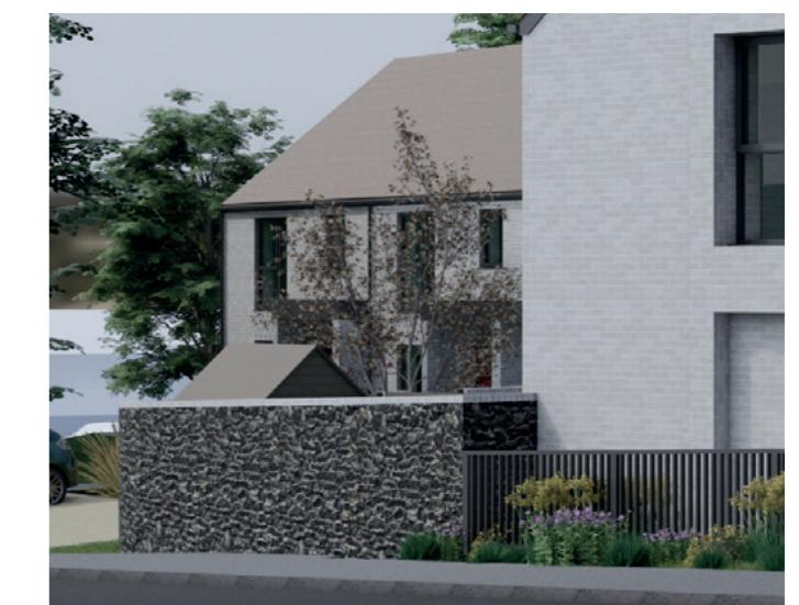
Excerpt from 3D model render showing re-purposed stone with facing brick capping
