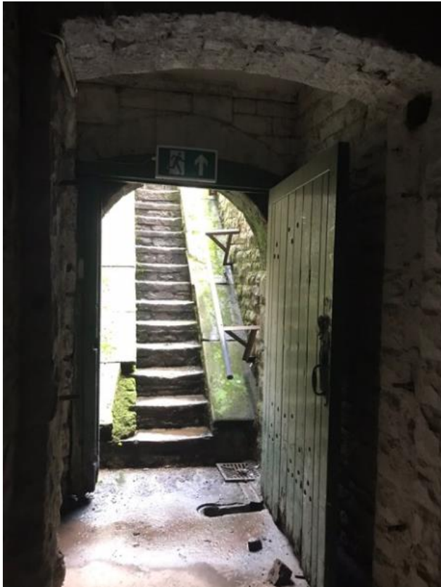
Cellar doorway from inside cellar, showing timber door since altered with a bat access slot added.
