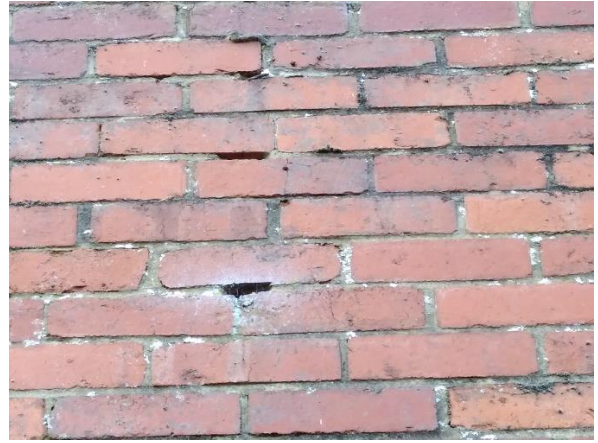
Figure 9 - Missing brickwork mortar on B1 eastern gable walls
