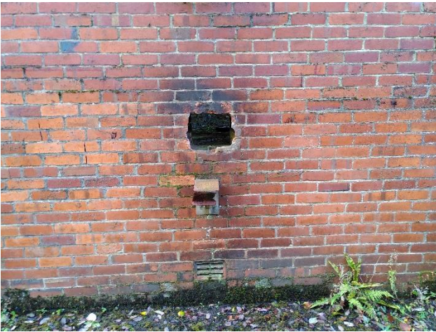
Figure 10 - Hole in the wall in B1 exposing cavity for winter hibernation
