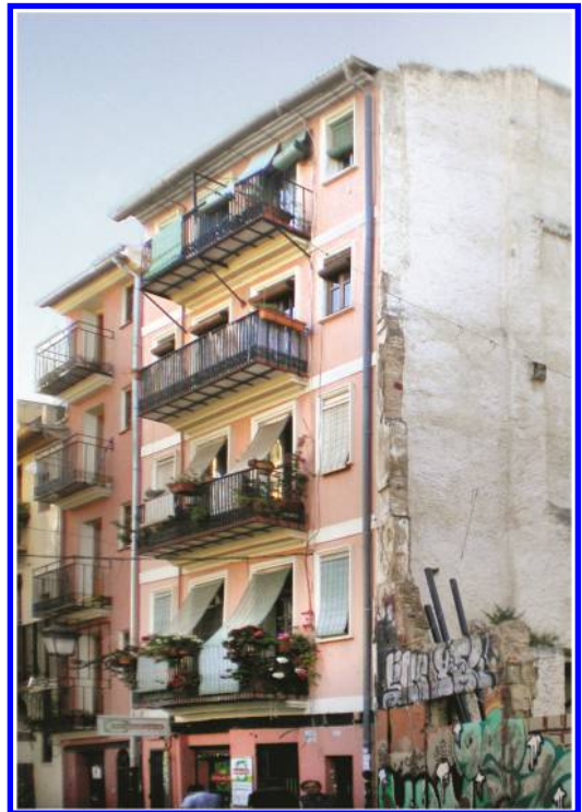
Figure 1. Mid-19th century building in the historic center of Valencia, Spain. Case study.
