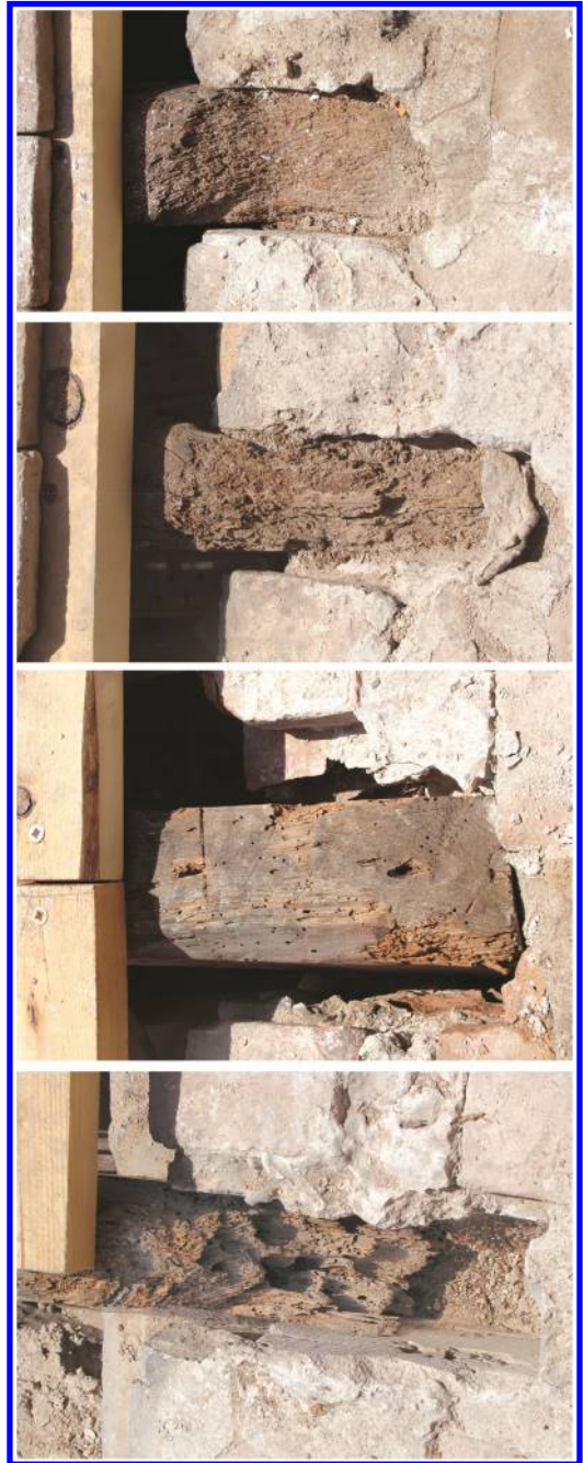
Figure 5. Rafters: V-19, V-20, V-21 and V-22.
