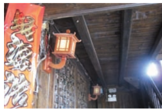
Figure 13. The wooden floors of the room.
