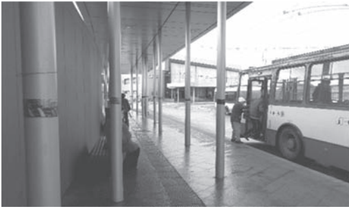
Figure 3. Columns intervening in the trolleybus stop area
