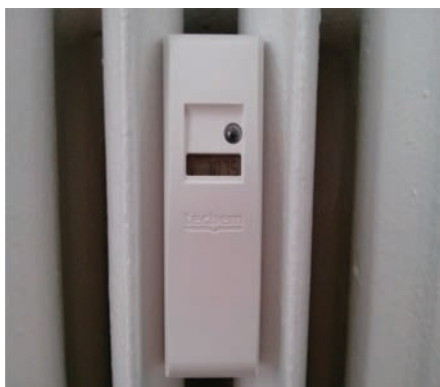
Figure 1. Example of heat cost allocator with radio data transmission.
