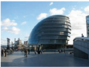
Figure 1. Full view of London City hall.
