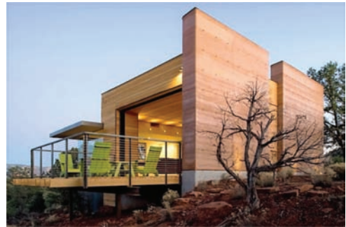
Figure 1. The perch, a rammed earth architecture project, Sedona Arizona, 2008, by courtesy of The Construction Zone.
