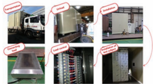
Figure 3. The process from transportation to the installation of the equipment.
