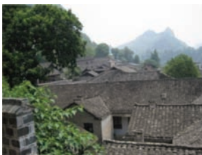
Figure 14. The tiles that the residences used.
