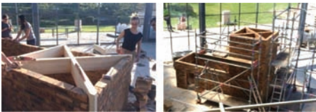
Figure 4. The process of construction of a Badgir.
