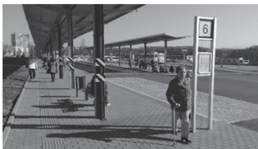
Figure 6. Columns with sufficient contrast marking.
