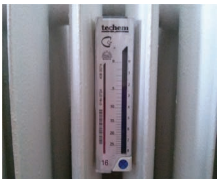
Figure 2. Example of heat cost allocator without radio data transmission.
