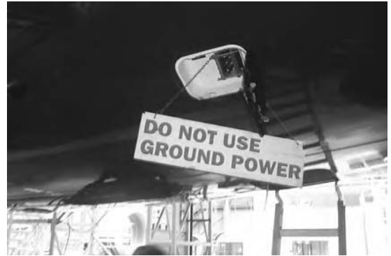
Figure 1.21 Ground power warning.
