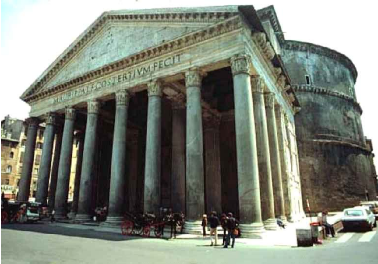
Fig.1. Pantheon in Rome. Concrete domical building 43 m high (115-125 A.D.)
