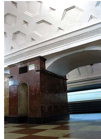
Fig.11. Moscow subway station "Red Gates". Monolithic concrete. The platform is ingrown 32.8 m (1935)
