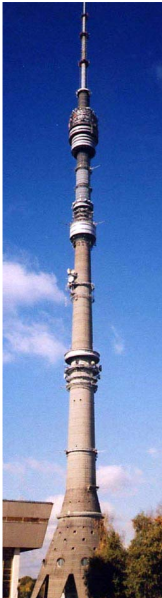
Fig. 14. Ostankino television tower, Moscow, more than 530 m high (1967)
