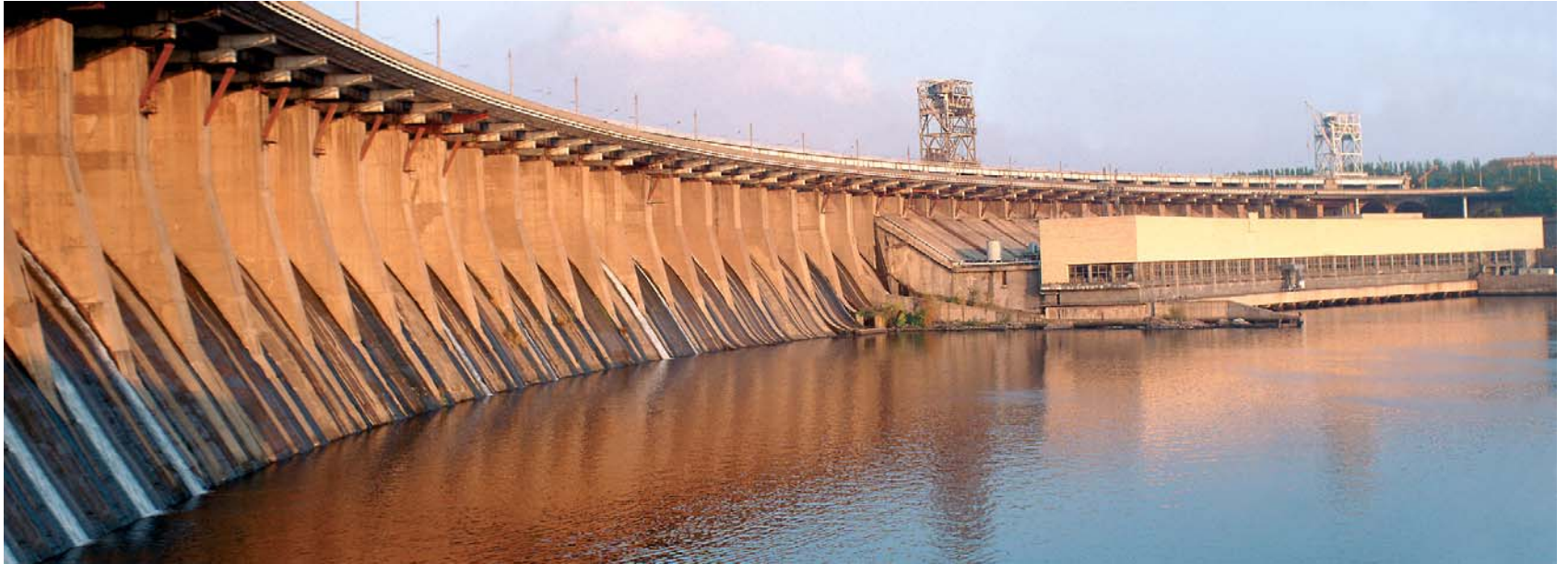
Fig.12. Concrete dam at Dnieper hydroelectric plant (1932)
