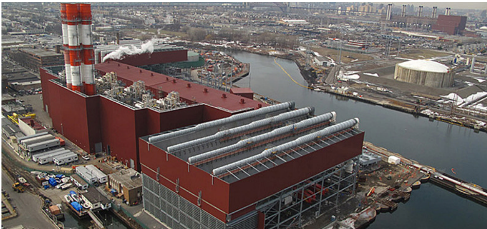
Figure 9.4 Power plant with an air-cooled condenser. Source: Reproduced by permission of the ATCO Group.
