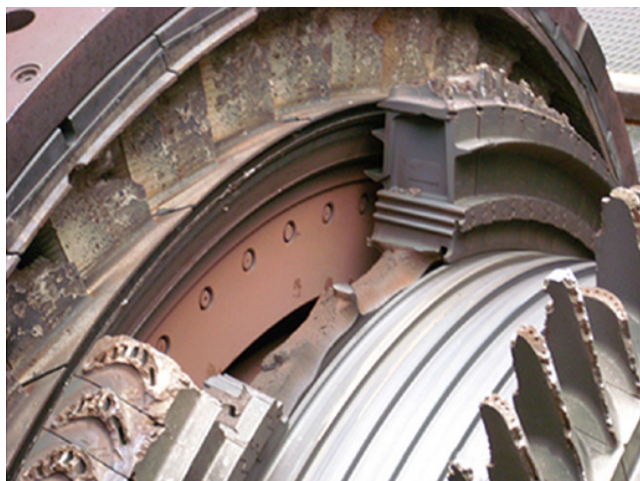
Figure 2.8 Failed turbine wheel and consequential damage. Source: Reproduced by permission of Phillips 66.
