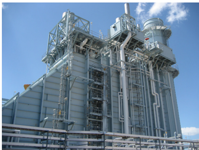
Figure 2.4 A photograph of an installed HRSG. Source: Reproduced by permission of Nooter/Eriksen.
