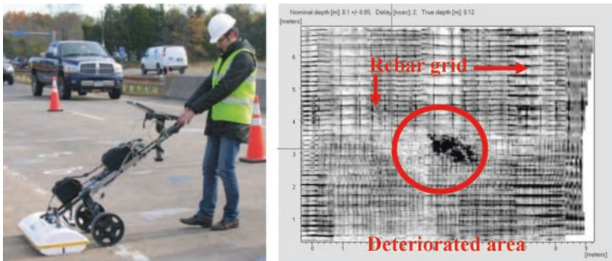
Fig. 4 GPR system RIS Hi-BrigHT specially designed for bridge deck surveying (left), visualisations of measured data at a depth of 10 cm with visible rebar grid and deteriorated area in the centre (right). Source IDS and (Alani et al. 2014)
