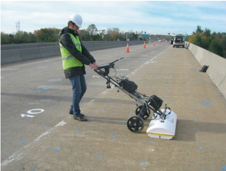
Fig. 13 Bridge deck survey with high resolution Ground Penetrating Radar (IDS HiBrightT)
