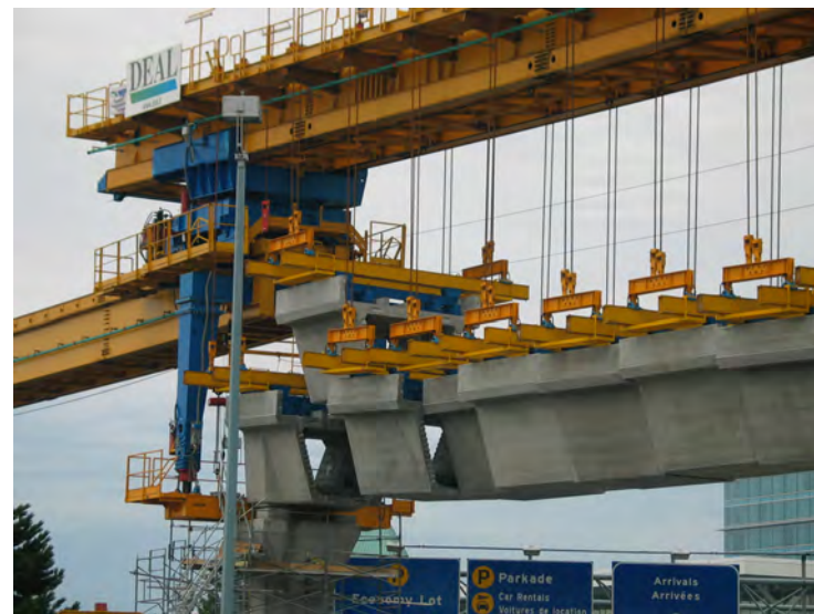
Figure 54.8: Erection of precast concrete bridge segments using an overhead erection girder.
