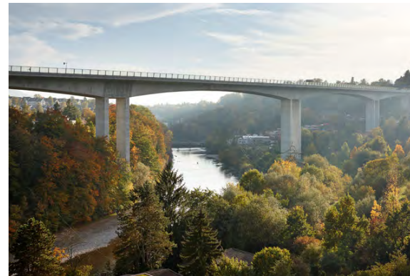
Figure 7.30: Photograph of the bridge depicted in the drawing of Figure 7.29. Photo: Ralph Feiner
