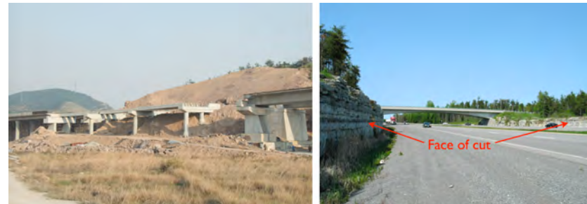
Figure 56.3: Examples of cuts used in highway construction
