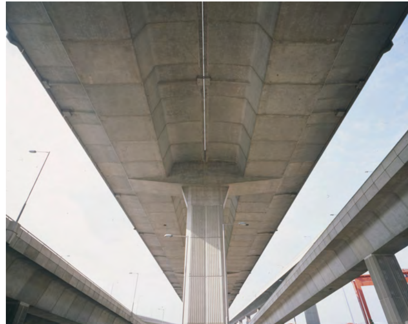
Figure 54.6: A precast segmental bridge in Hong Kong.
