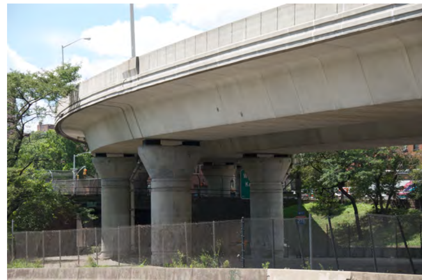
Figure 39.1: Photograph of the pier to be drawn
