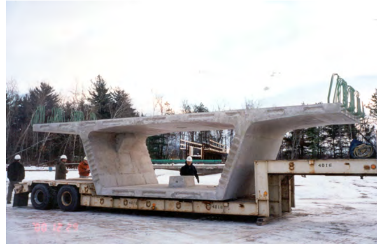
Figure 54.7: A precast concrete bridge segment.
