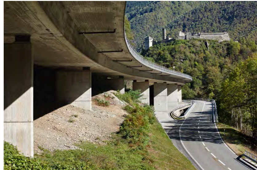
Figure 54.1: Pregorda Bridge, Switzerland. Design by Christian Menn. Photo by Ralph Feiner.
