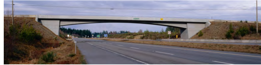
Figure 5.4: Royston Road Underpass, British Columbia. Design: Paul Gauvreau
