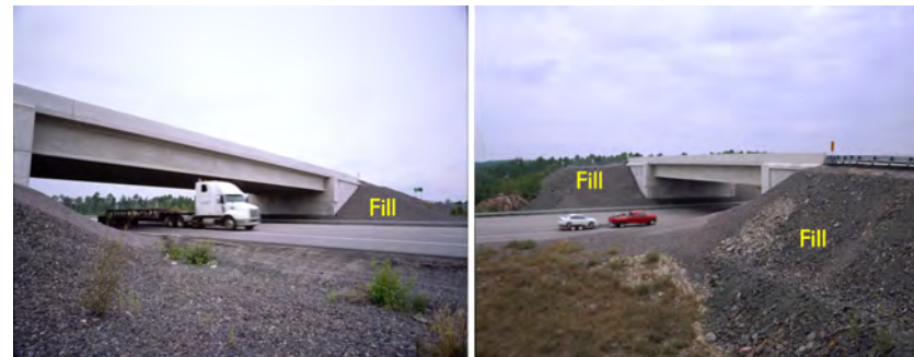
Figure 56.1: Fills used for the approaches to a highway overpass
