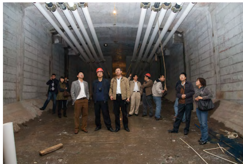
Figure 54.4: Interior of a single-cell box girder bridge.
