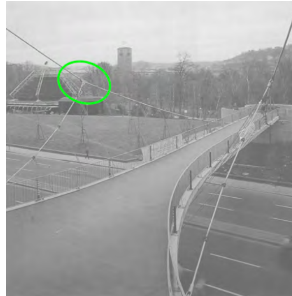
Figure 51.1: AutoCad Class 10: Cable connector to be dimensioned Bridge over the Neckarstrasse in Stuttgart, Germany. Design: Jörg Schlaich.
