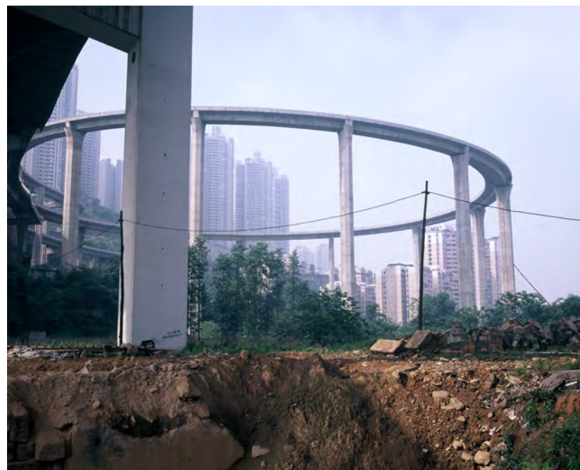
Figure 54.5: A curved single-cell box girder bridge in China.
