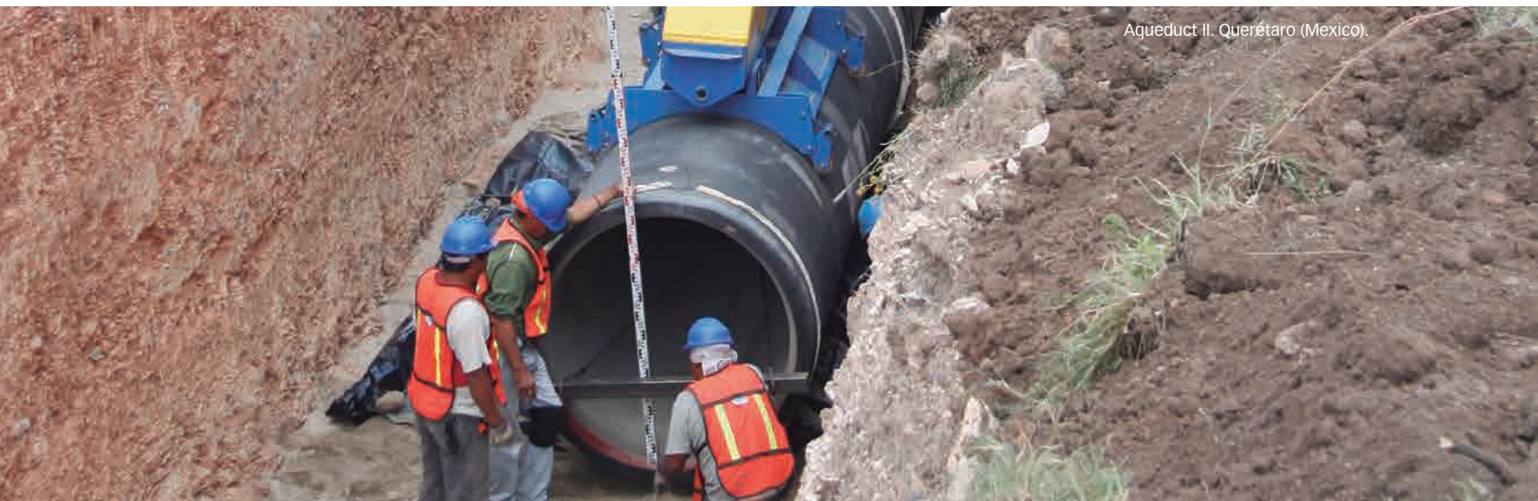
Navarra Canal (Spain).
