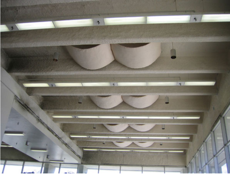
Figure B6.6 An exposed one-way joist system
