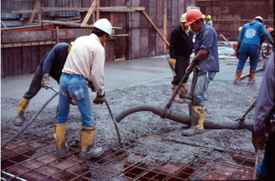
Figure B1.3 Concrete placement by pump
