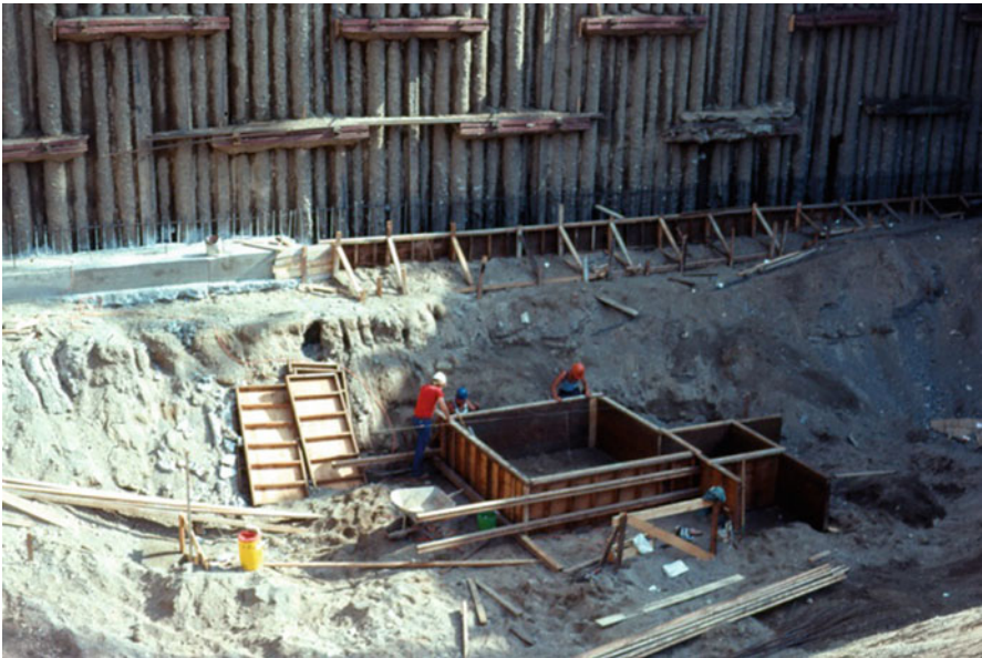
Figure B7.1 A large square spread footing under construction
