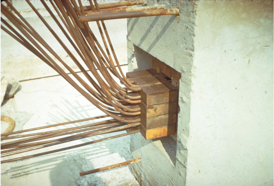
Figure B9.2 End anchor for a post-tensioned concrete beam Courtesy of the William G. Godden Collection, NISEE-PEER, University of California, Berkeley
