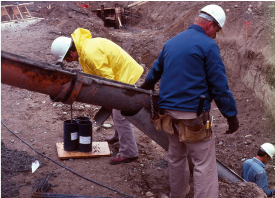
Figure B1.4 Concrete placement by chute and test cylinders in preparation
