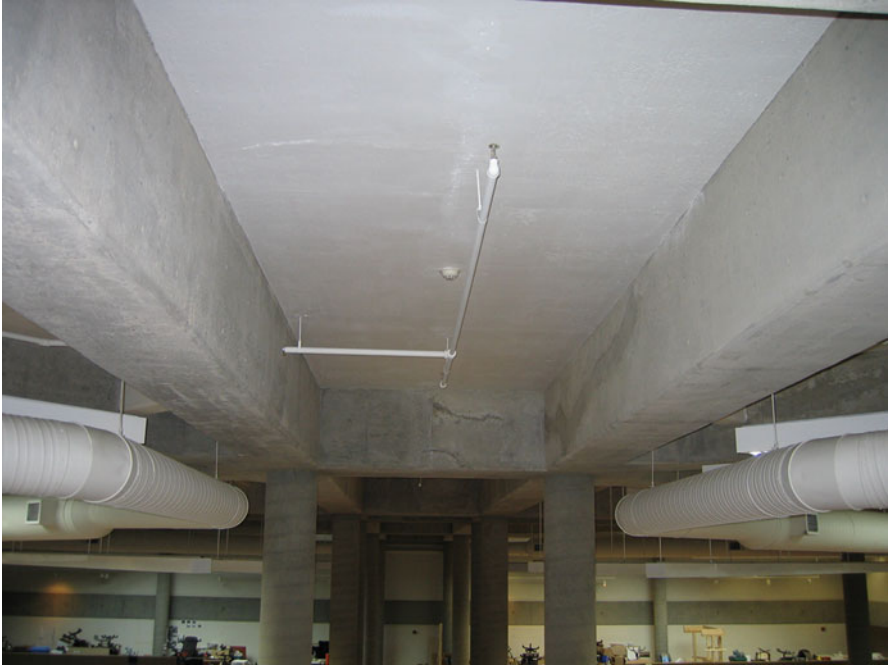
Figure B2.3 Beams supporting a one-way slab
