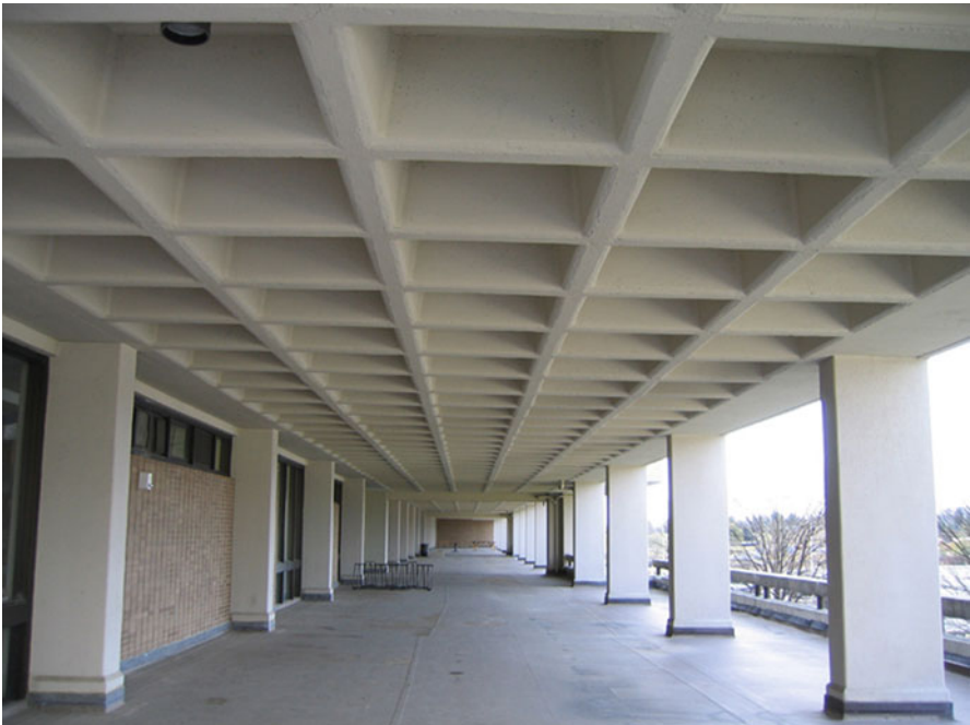
Figure B6.3 An exposed waffle slab floor system
