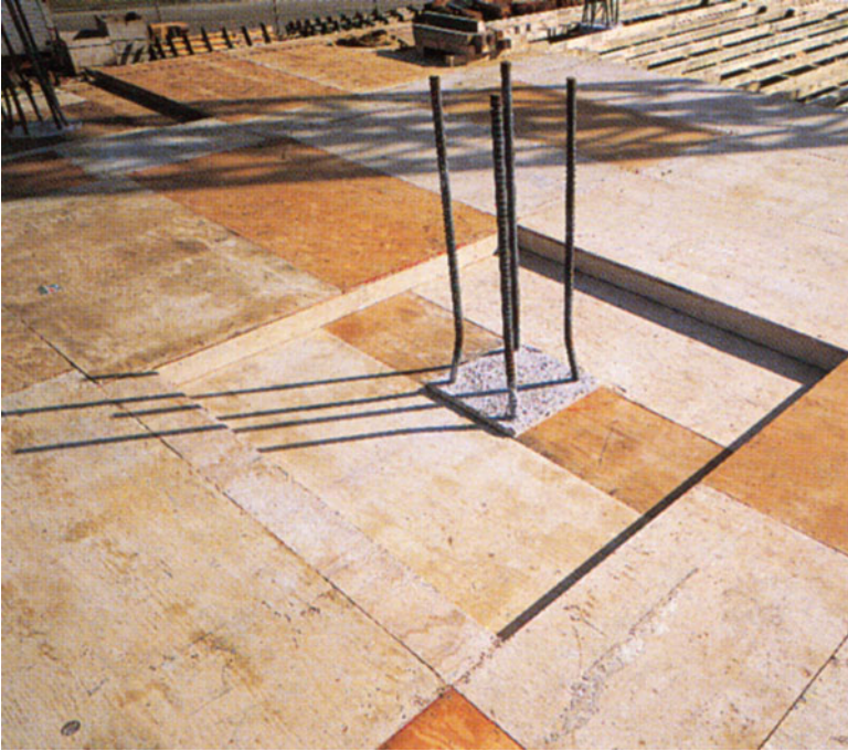
Figure B6.2 Forming for flat slab with drop panels
