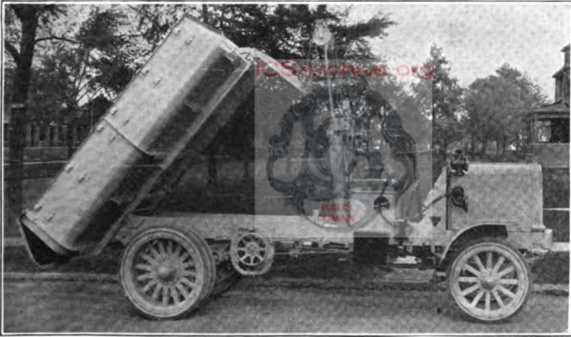
Fig. 351. Packard Truck with Hydraulic Tipping Gear
