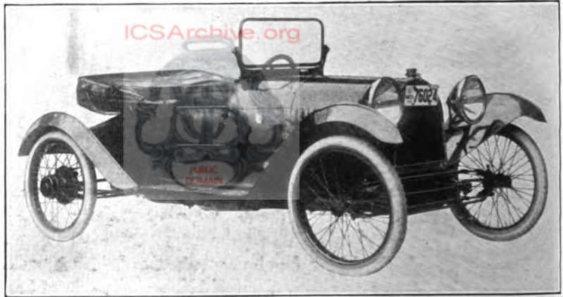
Fig. 31. Cornelian Light Car Courtesy of Blood Brothers Machine Company, Kalamazoo, Michigan
