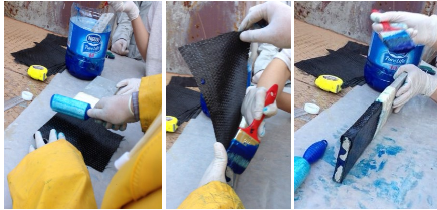
Figure 2.7: Application of CFRP on tensile test specimens.
