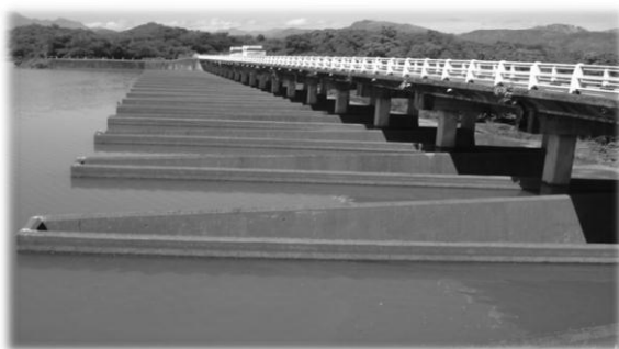
Figure 1: Labyrinth spillway at Loggal Oya
