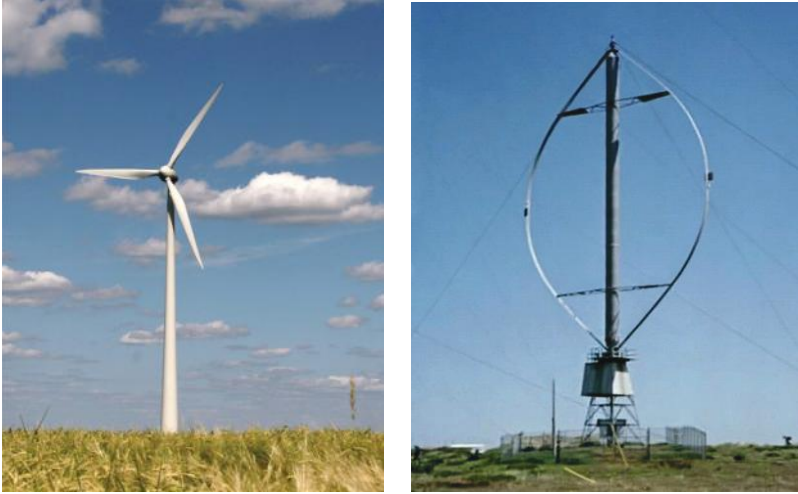
FIGURE 3.13 Two wind turbine designs. Left: A horizontal wind turbine (HAWT); and right: a vertical wind turbine (VAWT). Source: Left: http://en.wikipedia.org/wiki/File:Windenergy.jpg . Right: http://upload.wikimedia.org/wikipedia/commons/3/3c/Darrieus-windmill.jpg .
