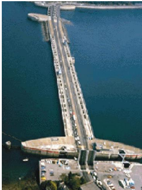
FIGURE 3.11 Rance Tidal Barrage, 240 MW power station, Brittany, France. Source: http://www.reuk.co.uk/La-Rance-Tidal-Power .
