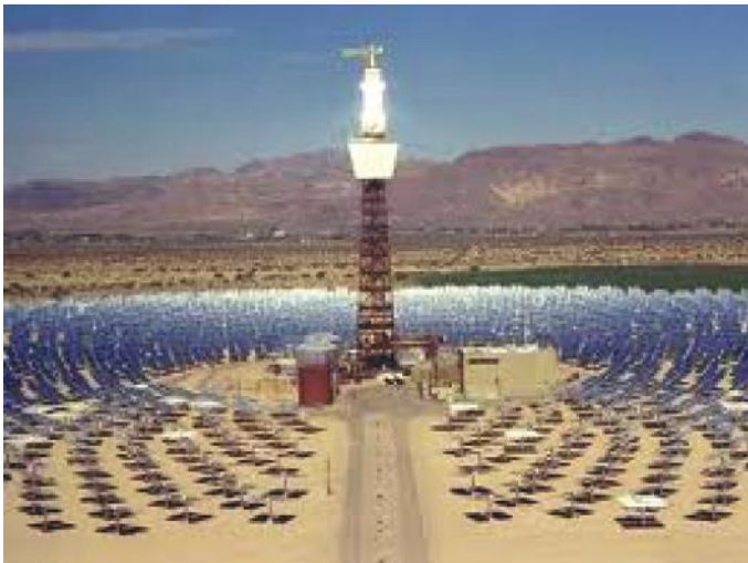
FIGURE 3.7 A solar thermal installation. Source: http://www.photovoltaic-solarenergy.com .
