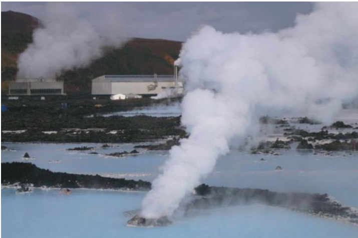
FIGURE 3.8 The Svartsengi Geothermal Power Station Source: http://en.wikipedia.org/wiki/Svartsengi_Power_Station .
