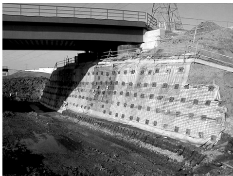
Figure 6.39 Soil-nailed wall along Midland Expressway, UK. (Image courtesy of Phi Group.)
