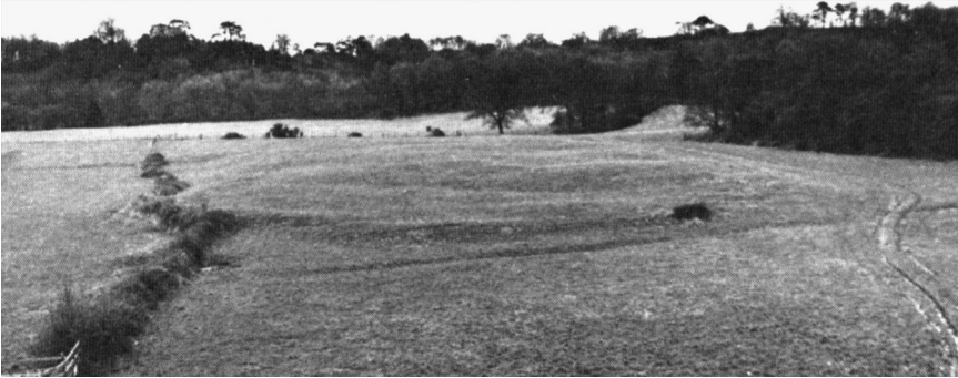
Figure 5.12 View from ground level of preexisting instability at Sevenoaks, Kent. (From Clayton, C.R.I. et al., Site Investigation , Second edition, Blackwell Science, 584 pp., 1995.)
