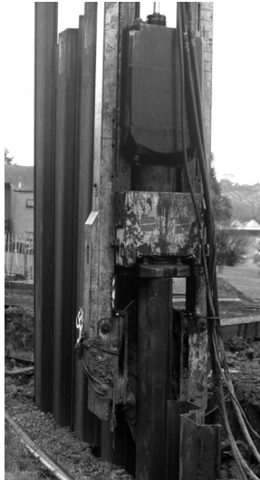
Figure 6.15 Driving Larssen steel sheet-piles.
