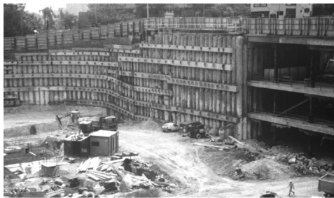
Figure 6.23 Anchored and propped bored pile retaining walls. Castle Mall, Norwich.
