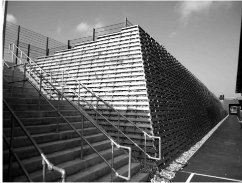
Figure 6.7 Large timber crib wall at University of Surrey.
