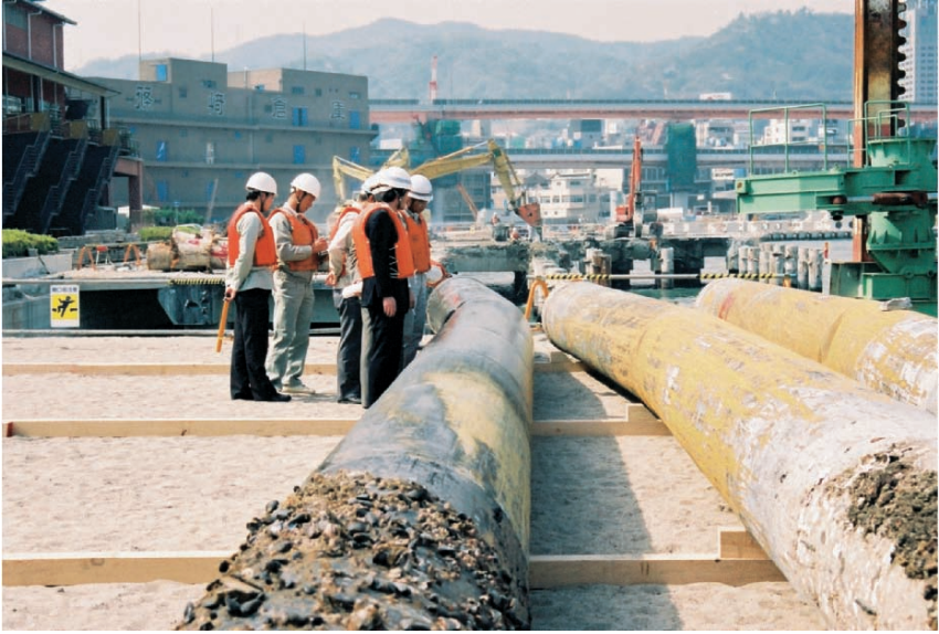
Fig. 13.15. Damage to steel piles for pile-supported-wharf in Kobe Port during 1995 Hyogoken-Nambu earthquake
