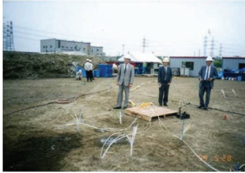
Fig. 15.20. Injection of colloidal silica liquid through multiple tubes into sandy ground
