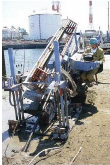
Fig. 15.23. Inclined drilling of borehole for grouting under existing structure
