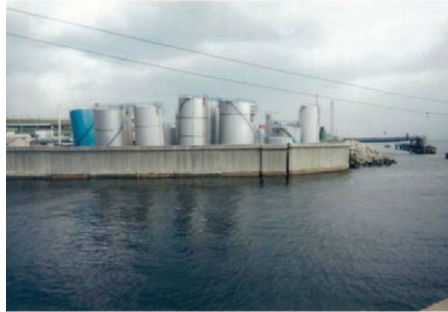
Fig. 15.17. Distortion of liquid storage tanks due to subsoil liquefaction (Kobe, 1995)
