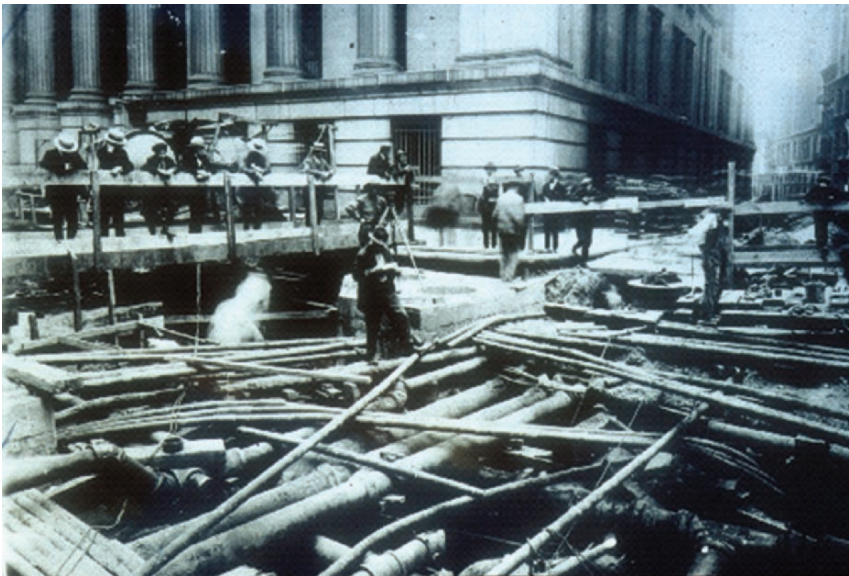
Fig. 17.1. Underground infrastructure at Wall and Williams Streets in New York City, 1917
