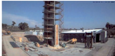
(b) 7-Storey Shear building model on shake table
