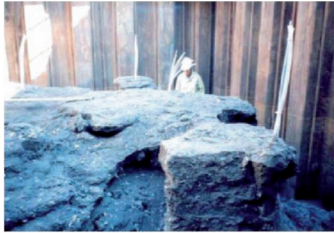
Fig. 15.21. Excavation of soil mass as solidified by silica grouting
