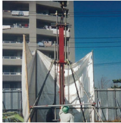
Fig. 15.49. Portable equipment for percussive penetration of screen pipe
