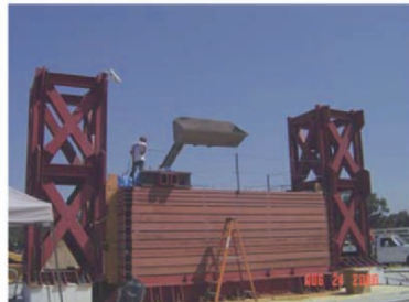
(d) Close-up of soil container on shake table during Model construction
