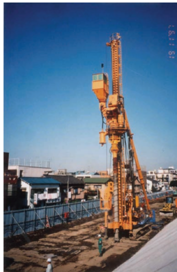
Fig. 15.39. Construction of gravel drain (Fudo-Tetra Inc.)
