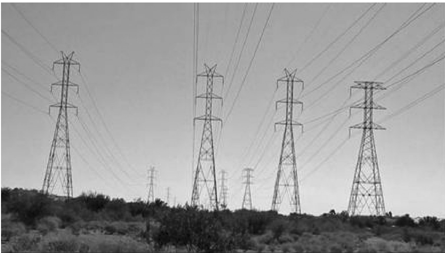
FIGURE 19.3 Transmission line corridor.
