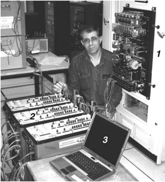
FIGURE 13.44 Testing of distance relay LZ-31 type by means of transient simulator 1 — Relay LZ-31; 2 — three-phase power simulator DOBLE-2500; 3 — PC with transient file, previously loaded from fault recorder.
