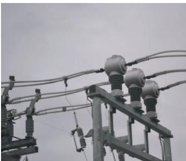
FIGURE 2.24 Current transformer.
