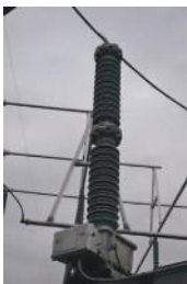
FIGURE 2.21 Voltage dividers.
