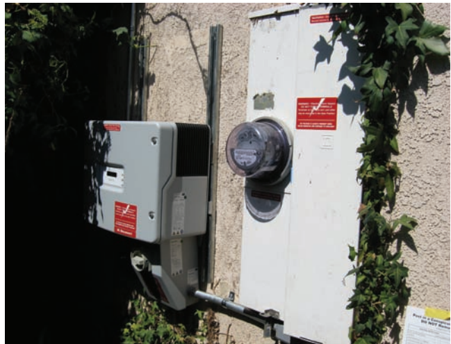
FIGURE 33-4 A residential utility-interactive inverter. (Delmar/Cengage Learning)
