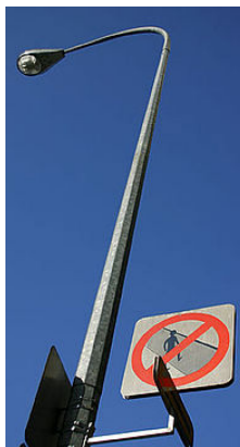
A street lamp in Singapore showing the characteristic spangle of hot-dip galvanization.
