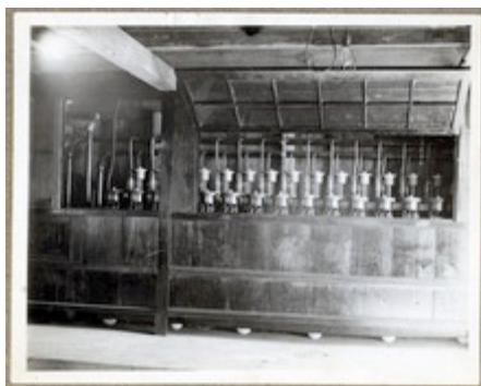
Electrolytic cells for hydrogen production, Fixed Nitrogen Research Laboratory, ca.1930s
