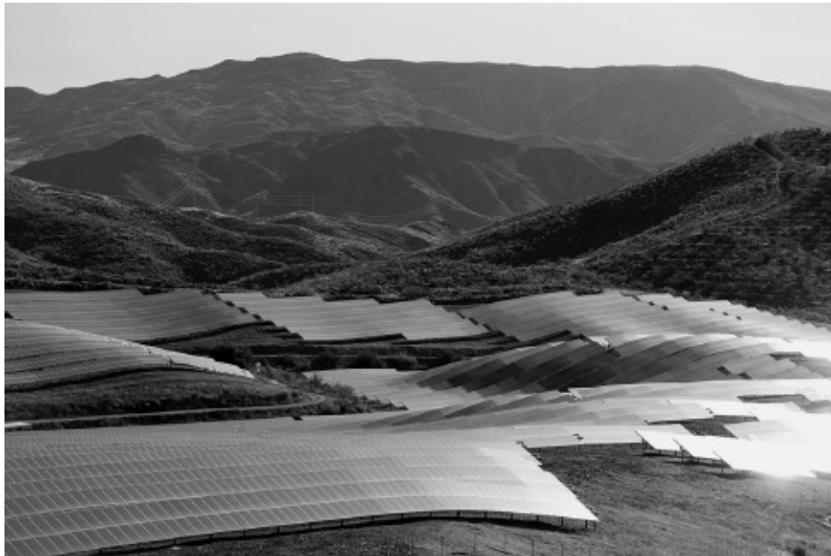
Figure 5.16 Lucaneina de las Torres photovoltaic power plant in Spanish Andalusia (Corbis).
