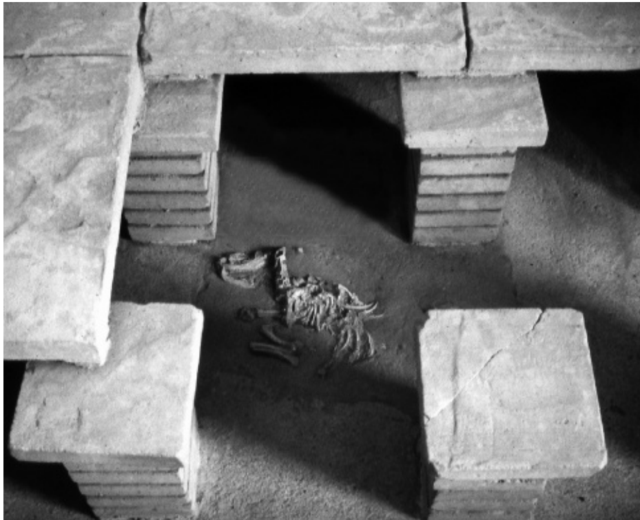
Figure 4.16 Part of a Roman hypocaust (with the skeleton of a dog killed by fumes) displayed at Homburg-Schwarzenacker Roman Museum in Saarland. Photograph courtesy of Barbara F. McManus.
