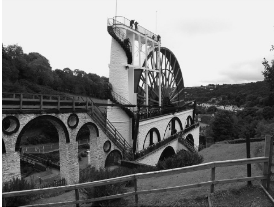
Figure 4.11 The Great Laxey waterwheel after restoration (Corbis).
