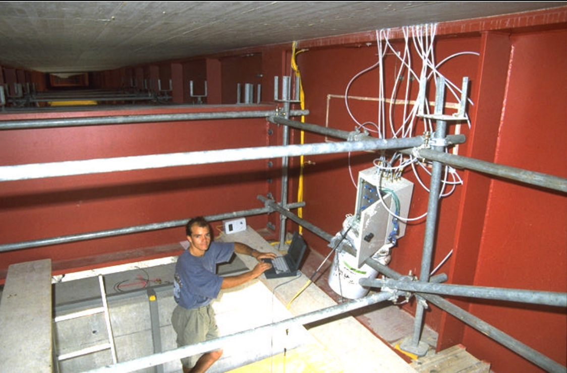
Figure 8.16. The Venoge highway bridge near Lausanne. Typical measurement session.
