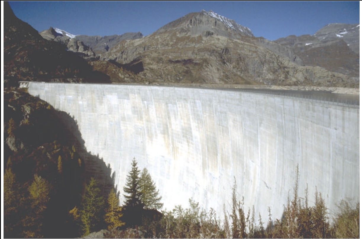
Figure 8.26. The Emosson dam.
