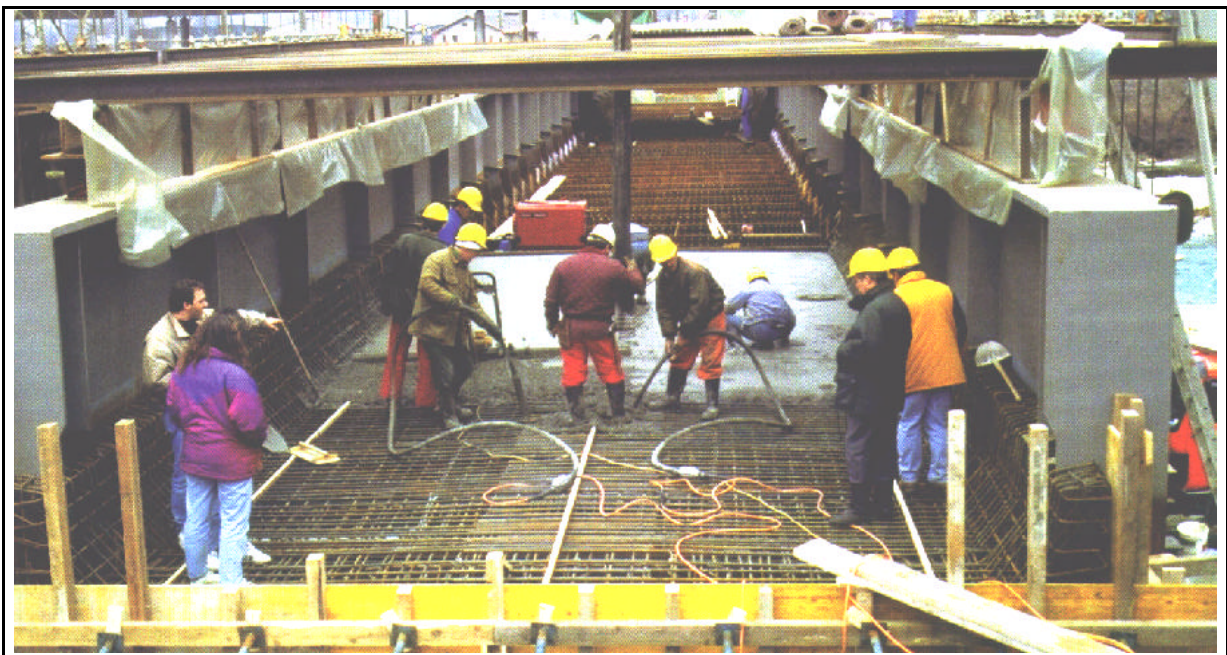
Figure 8.18. The Moesa railway bridge near Bellinzona.
