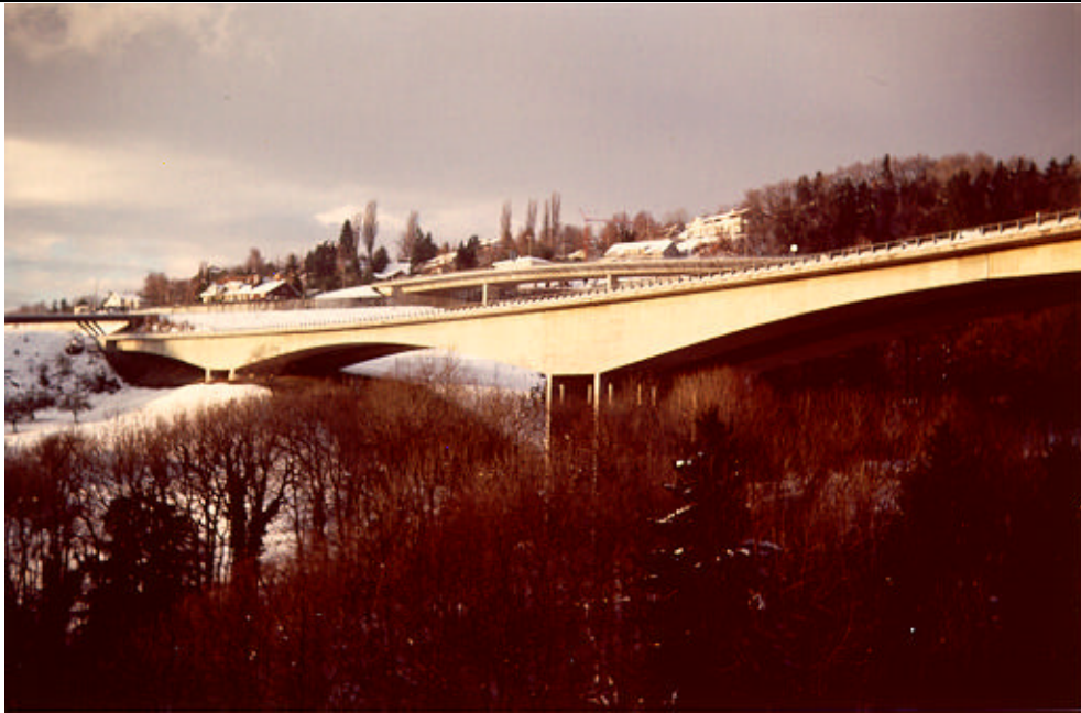
Figure 8.24. The Lutrive Bridge
