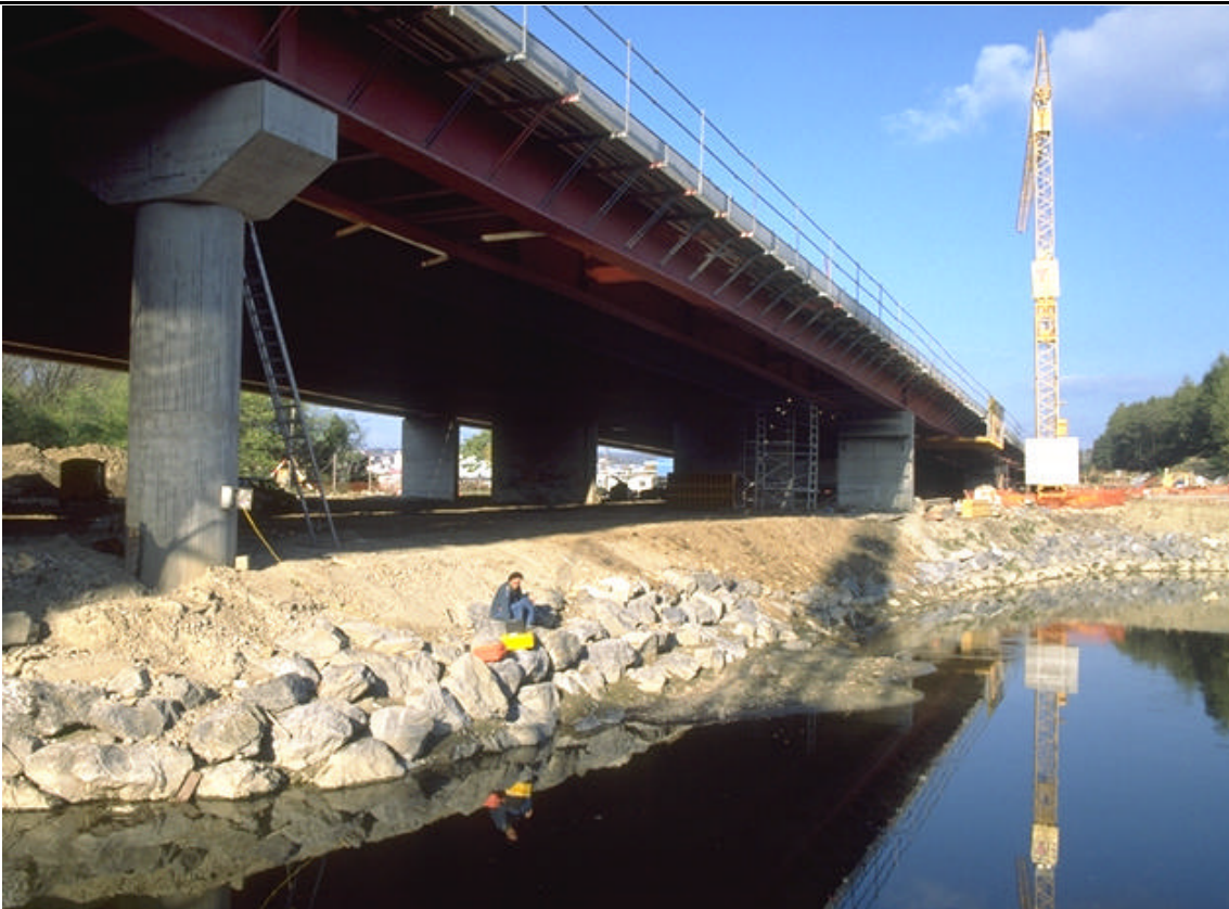
Figure 8.15. The Venoge highway bridge near Lausanne. General view.
