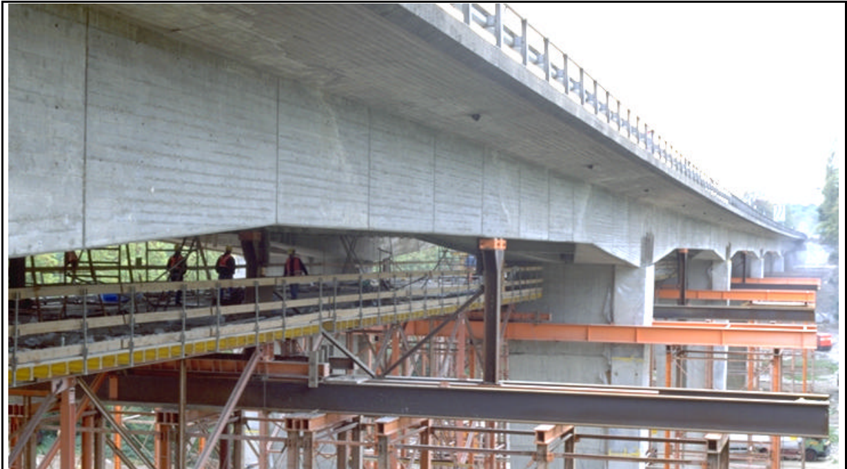
Figure 8.20. The Versoix highway bridge.
