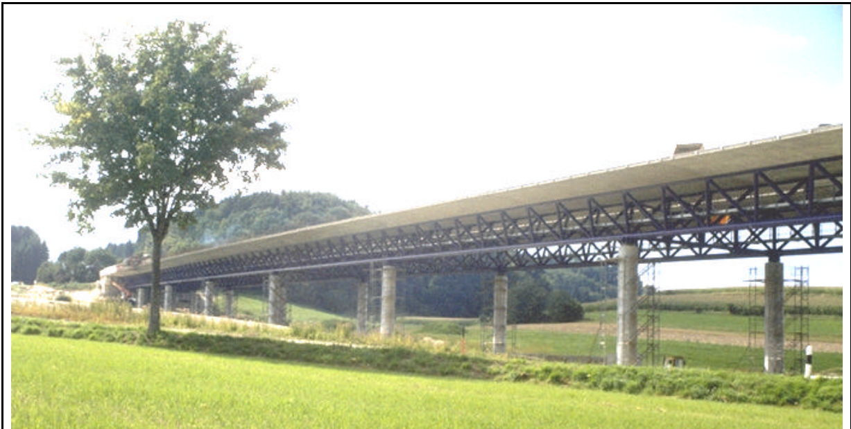
Figure 8.22. The Lully viaduct
