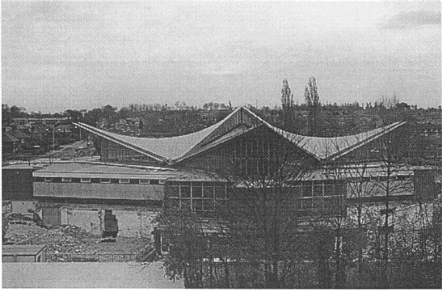
Figure 3. Hyperbolic-paraboloid shell roof.
