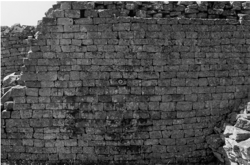
Figure 4.1 Dry stone masonry at Great Zimbabwe.
