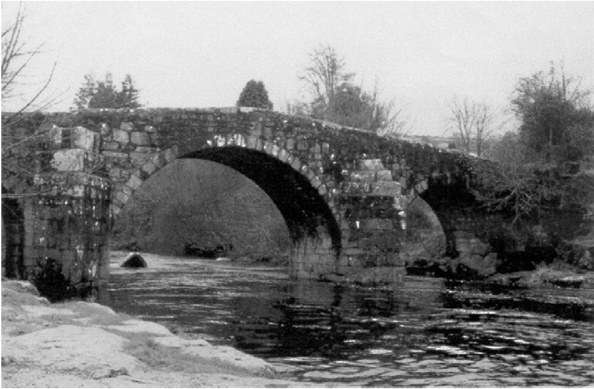
Figure 3.31 A masonry arch bridge.
