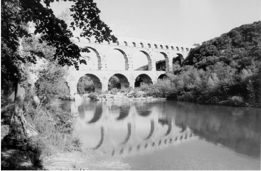
Figure 4.2 Pont du Gard – a Roman aqueduct showing semicircular arches.
