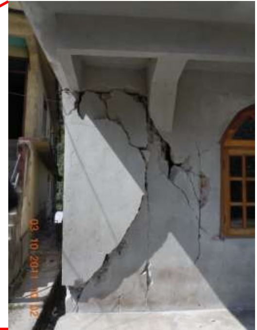
Unsupported wall on cantilever projection
