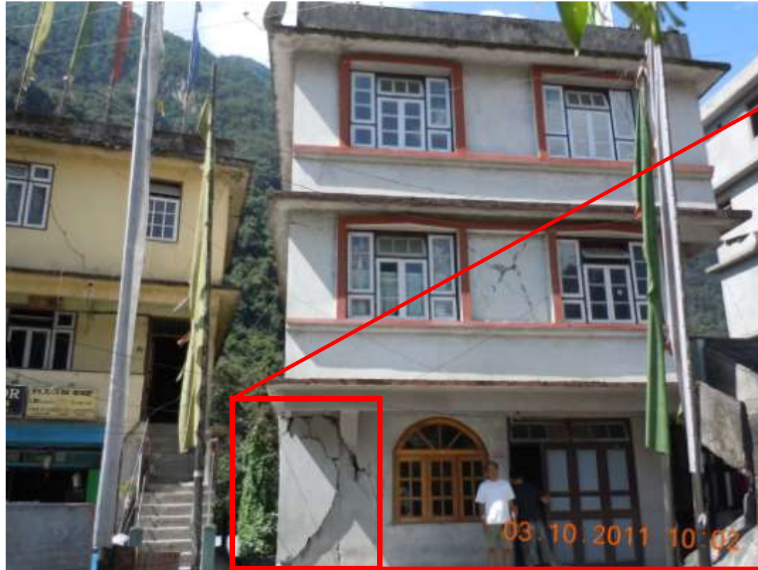
Unsupported wall on cantilever projection
