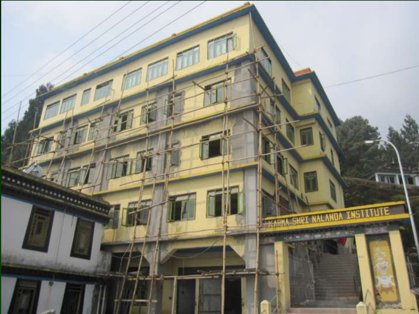
Retrofitting of Damaged RC Columns, Rumtek
