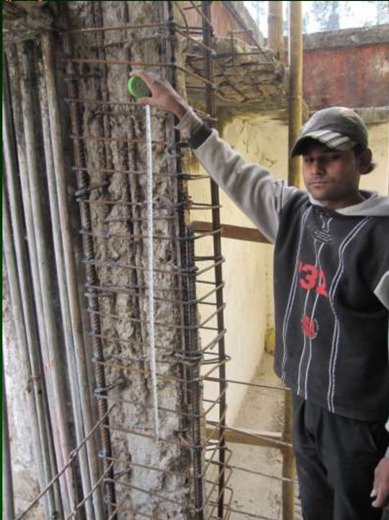
Retrofitting of Damaged RC Columns, Rumtek
