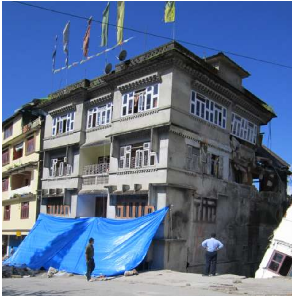
Demolition of 9- storey building at Balwakhani
