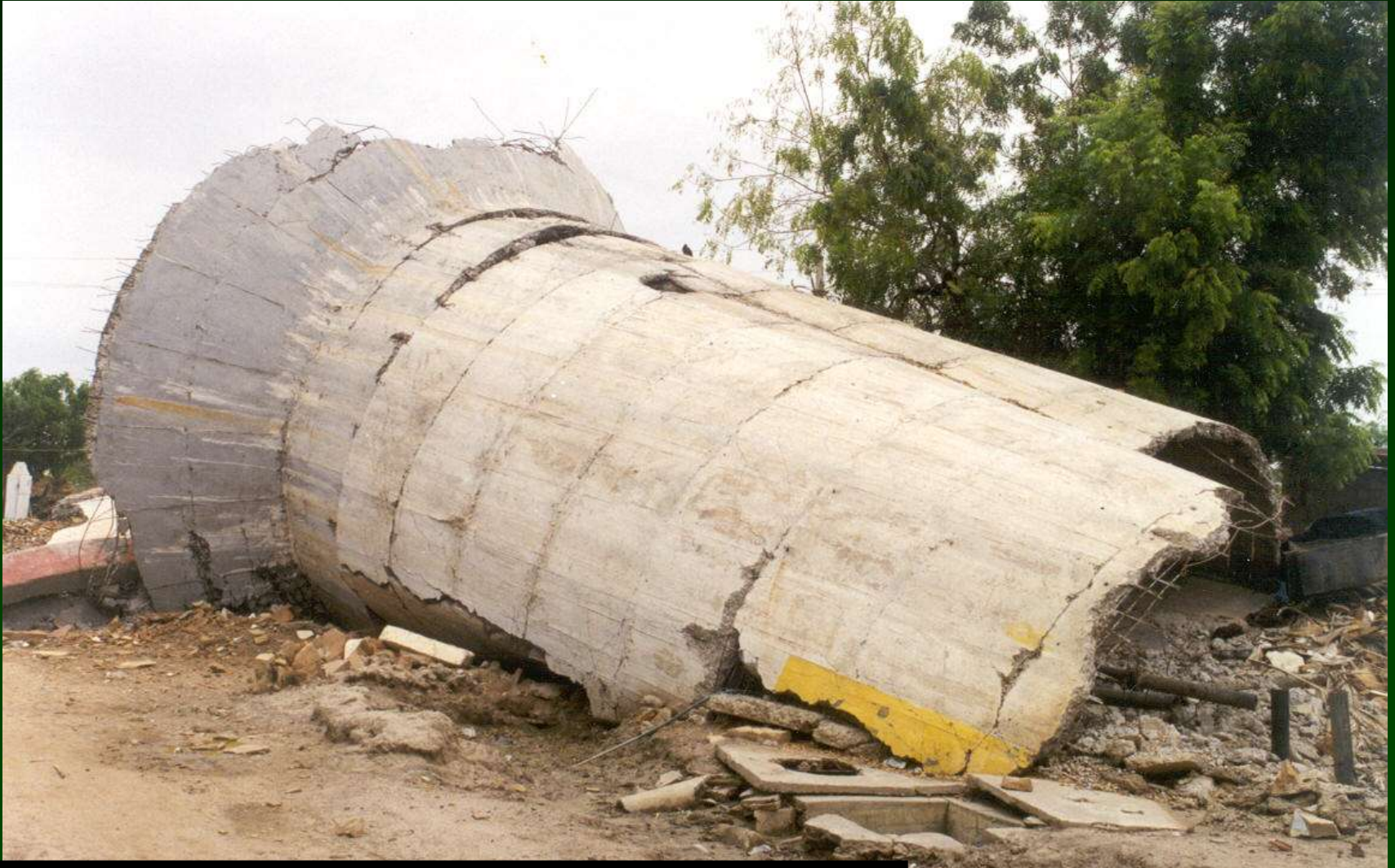
Shaft Supported Tank at Chobari
