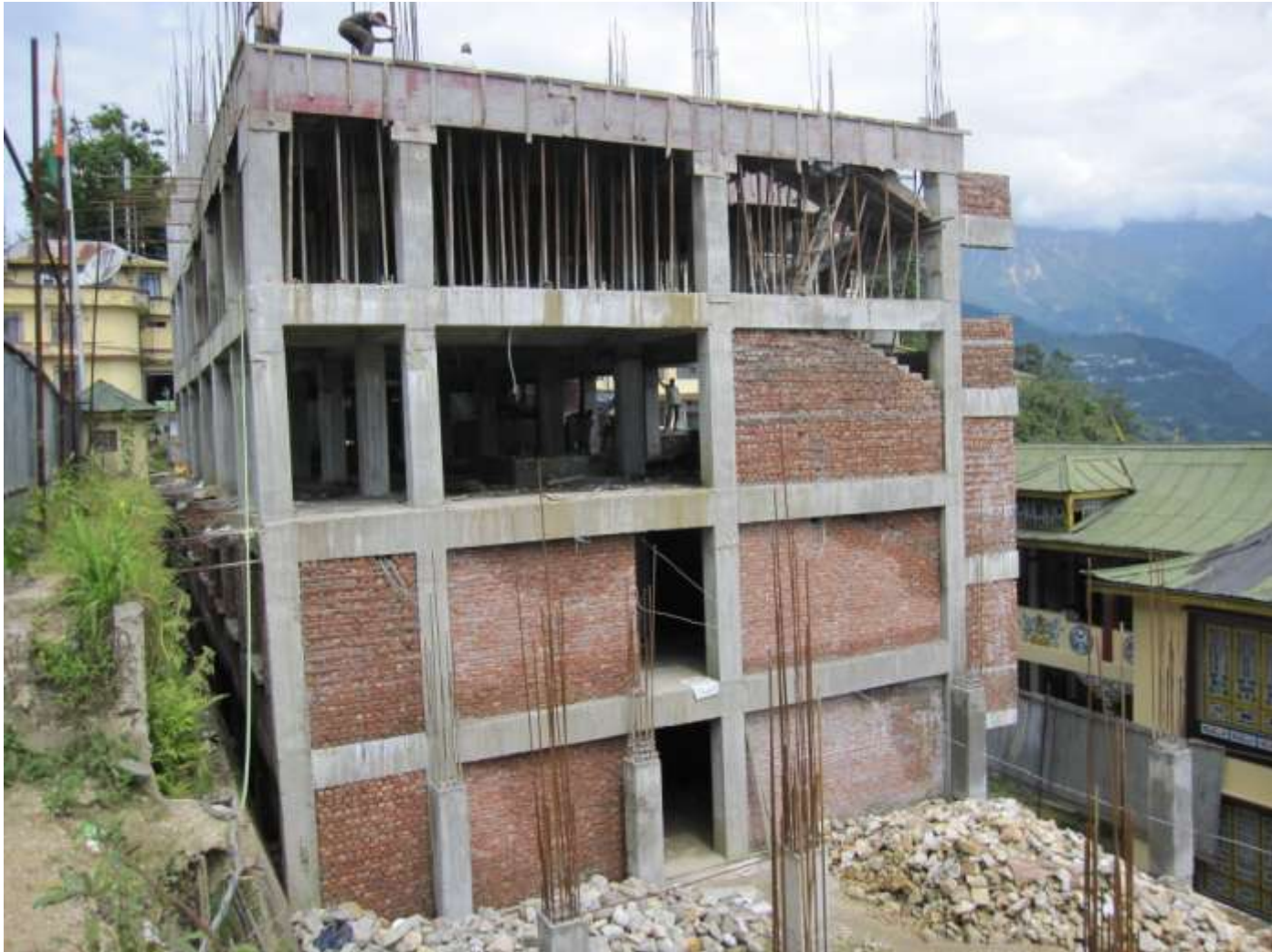
Construction of Annexe to Tashiling Secretariat, Gangtok
