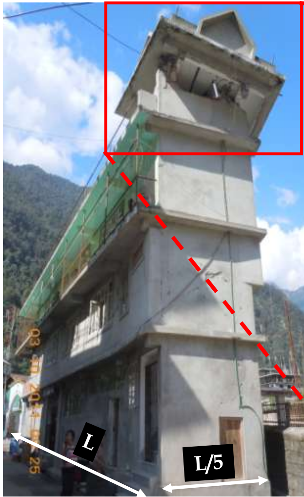
Collapse of appendage in a 3 storey building at Chungthang
