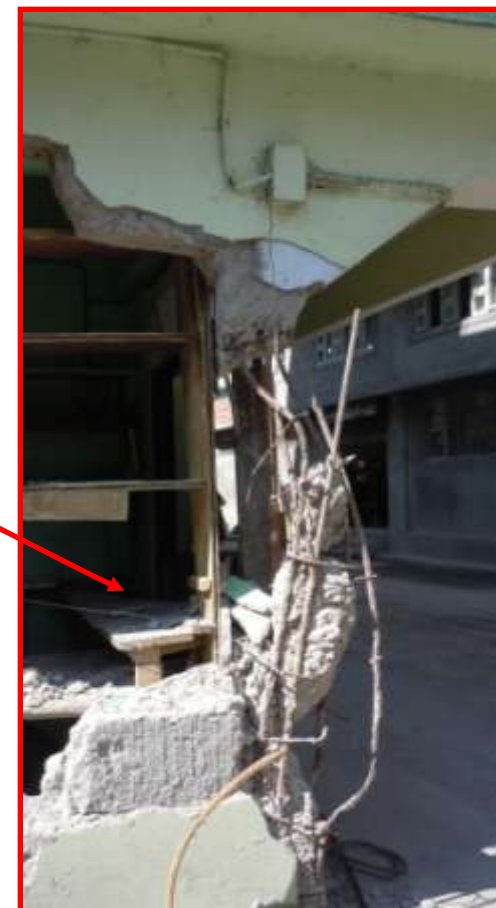
Improper Splicing
