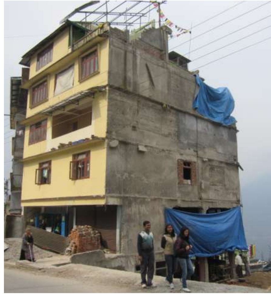
Retrofitting of the adjacent building
