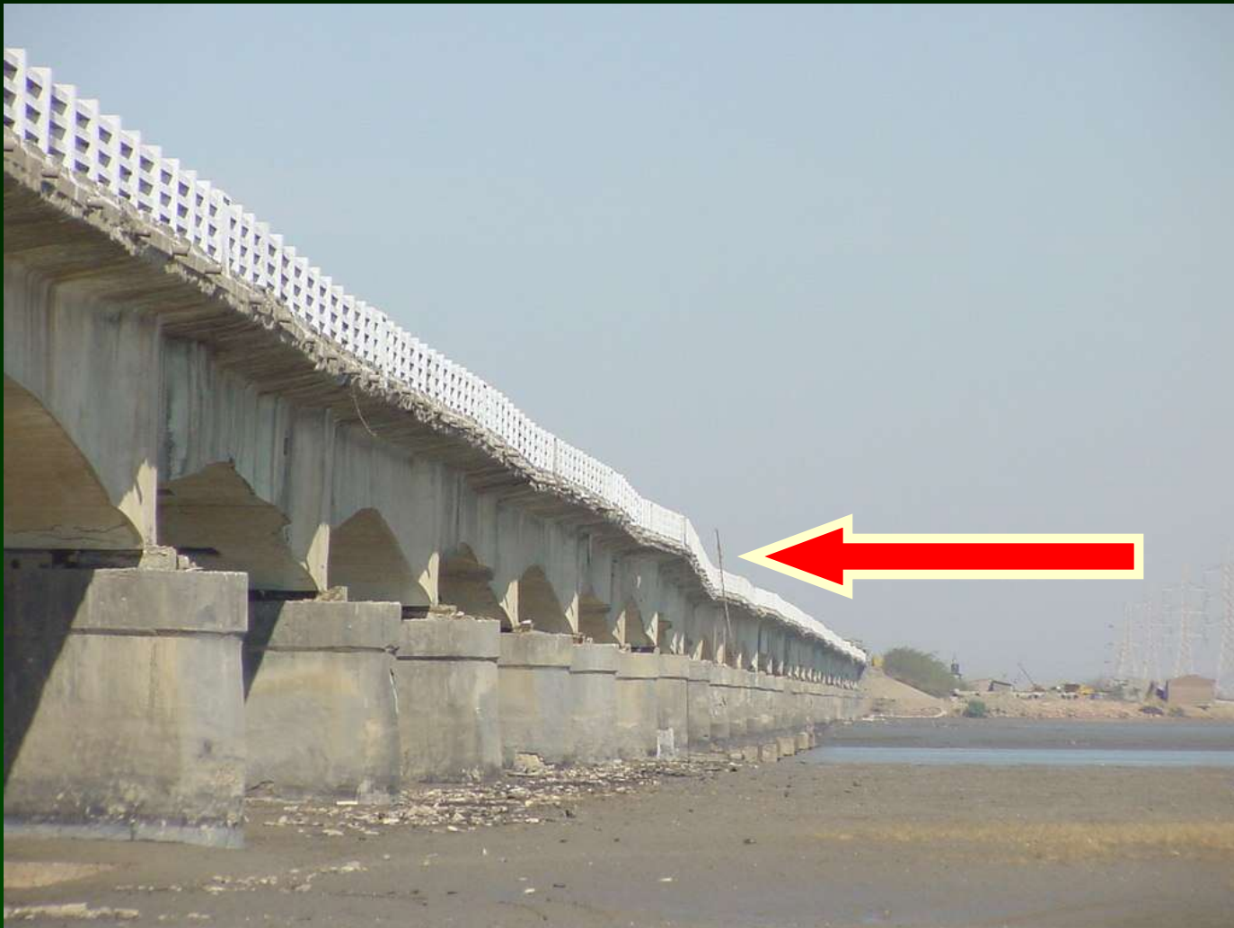
The Old Surajbadi Highway Bridge Balanced Cantilever Multi-Span Concrete Bridge
