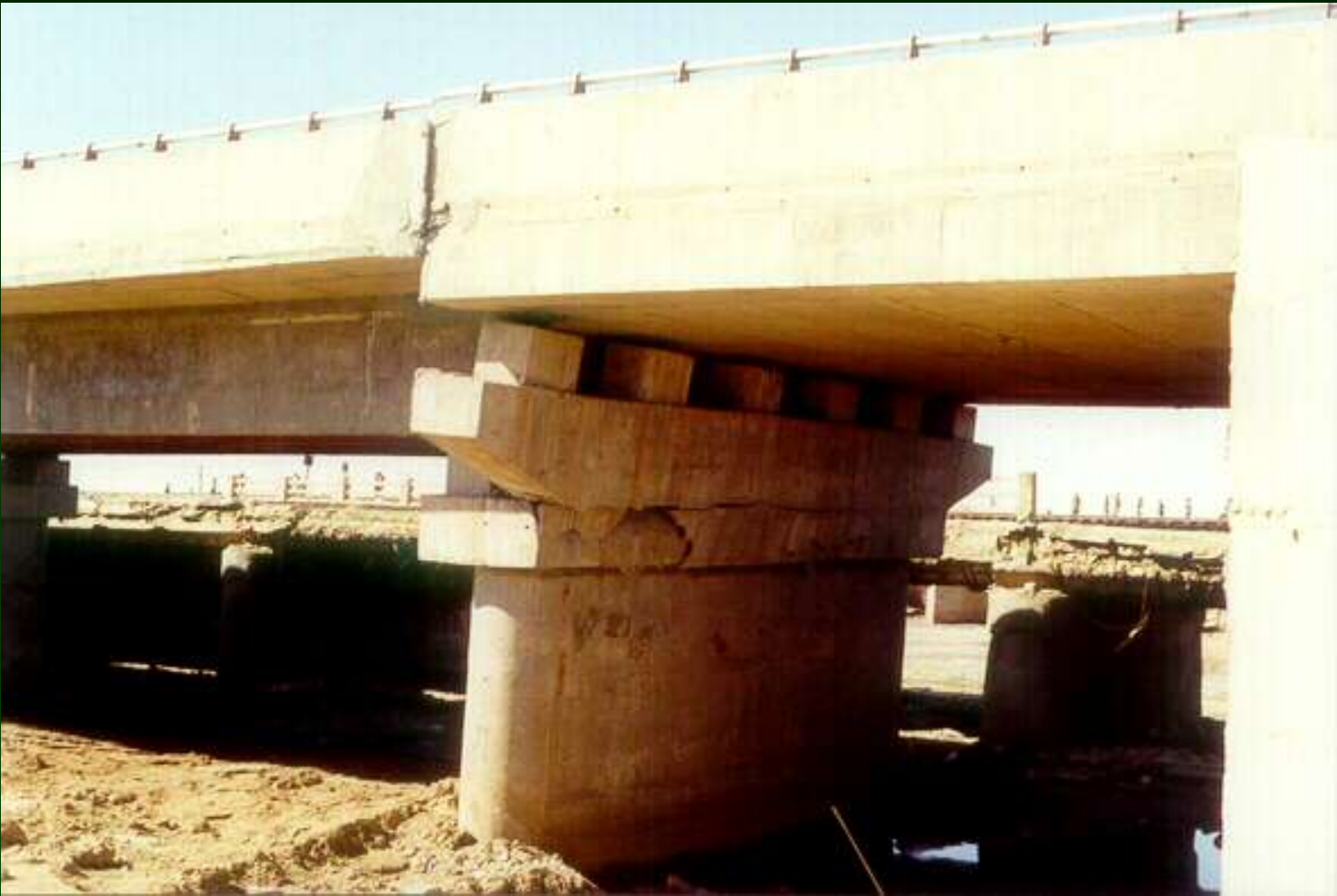
Modern RC Highway Bridge at Vondh Poor Configuration of bed blocks
