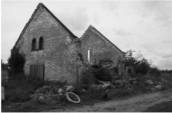
Fig. 10. The cattle-shed (photo 2009) [Source: State Inspection for Heritage Protection. Monument Documentation Center]
