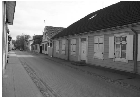
Fig. 3. Bauska. The reconstruction of the historic wooden building and the street cover [Source: photo by the author, 2012]
