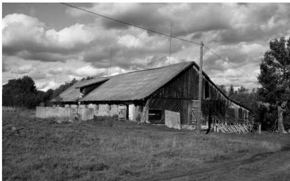
Fig. 12. The cattle-shed near the servants' house [Source: photo by the author, 2009]
