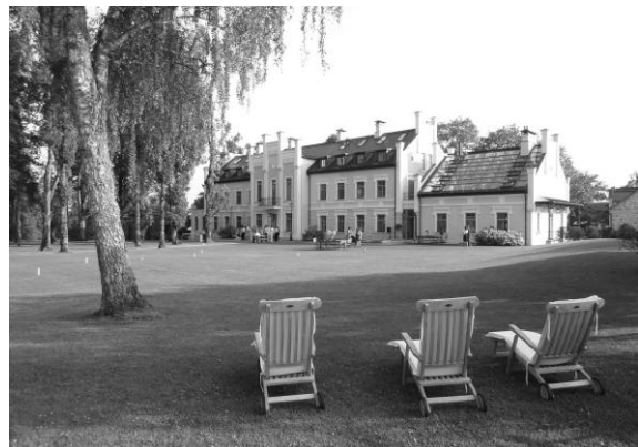
Fig. 10. The restored Rūmene Manor and the perfectly attended park have become a benchmark for the attitude full of understanding in the preservation of the historical cultural environment [Source: photo by O. Spārītis, 2012]
