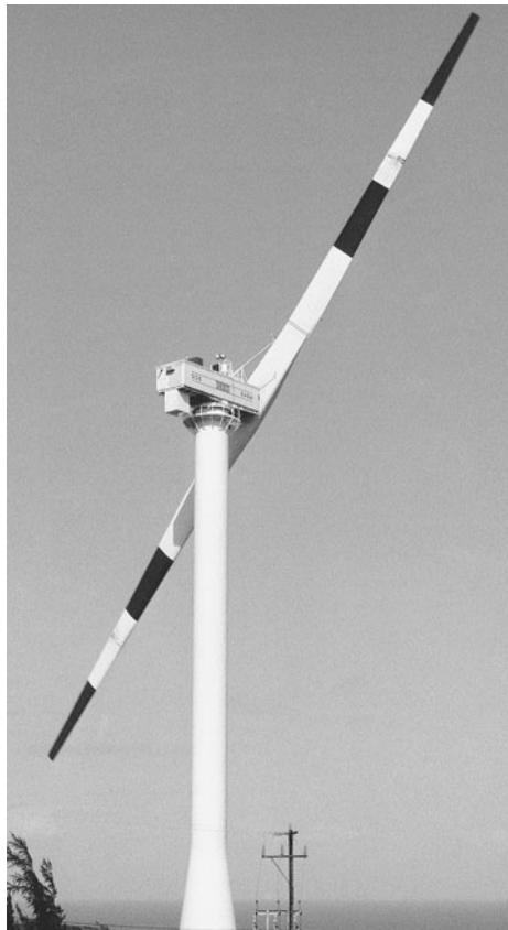
Figure 9.1 Large horizontal-axis wind turbine in operation on the Hawaiian island of Oahu. The blade has a tip-to-tip span of 98 m. (Photo courtesy of the NASA Lewis Research Center, Cleveland, OH.)
