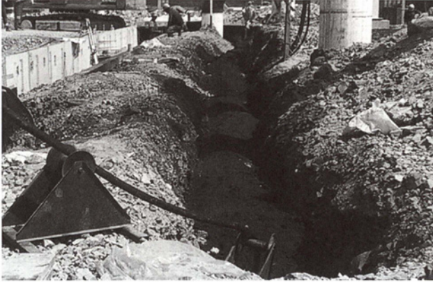
Laying of flexible anode
