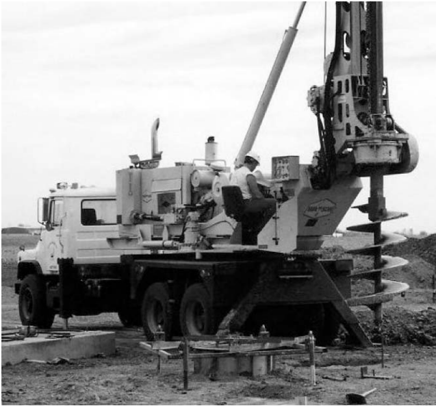
Figure 3.26 Watson 2100 truck-mounted auger drill.
