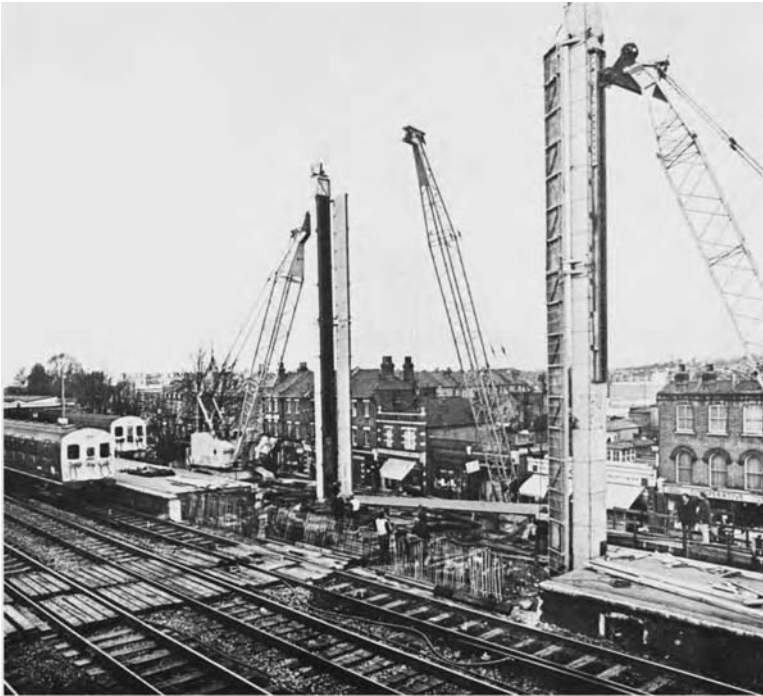
Figure 3.19 Noise-abatement tower used for 'Hush piling' system.
