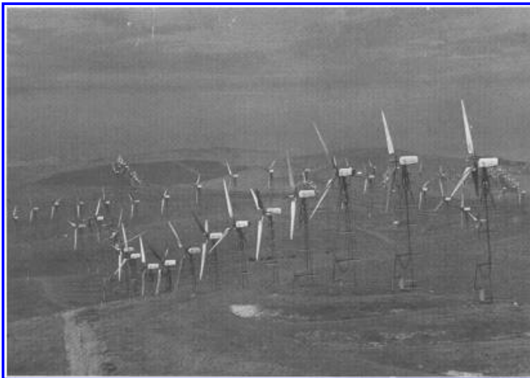
Fig. 5.3. Californian wind farm (17 m diameter, 100 kW WT, US Windpower Inc.).
