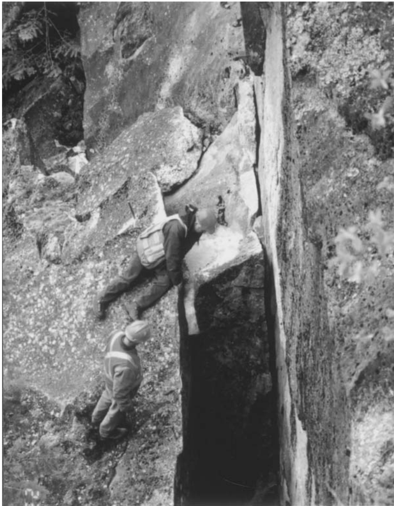
Figure 6.7 A tension crack behind a sliding rock mass in which significant horizontal displacement has occurred (above Kooteney Lake, British Columbia).
