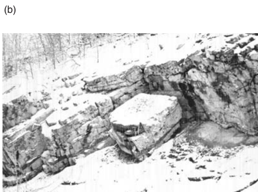
Figure 4.2 Plane failure on continuous bedding plane dipping out of the slope (strong, blocky limestone, Crowsnest Pass, Alberta, Canada).
