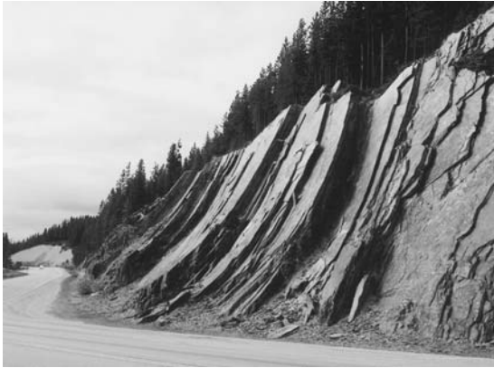
Figure 1.3 Cut face coincident with continuous, low friction bedding planes in shale on Trans Canada Highway near Lake Louise, Alberta. (Photograph by A. J. Morris.)
