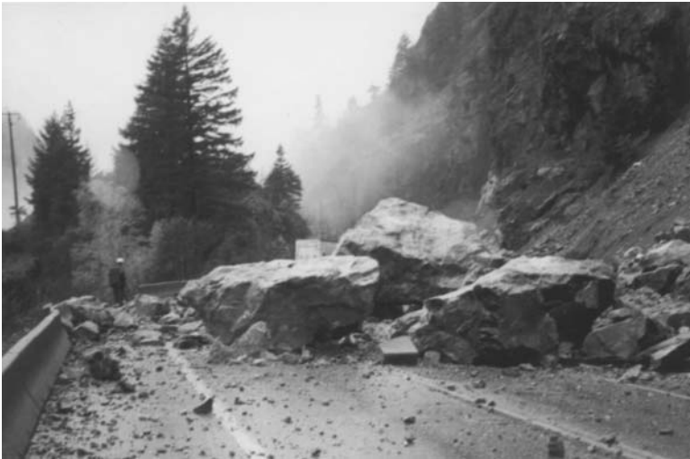
Figure 12.1 Highway closure caused by rock fall in very strong, blocky granite from a height of about 300 m.
