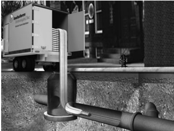
10.4 CIPP winch-in-place installation method (courtesy of Insituform Technologies).
