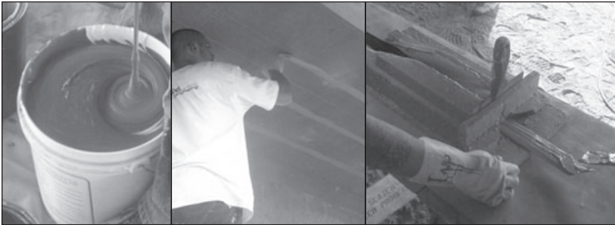
4.3 Mixing and application of epoxy adhesive.
