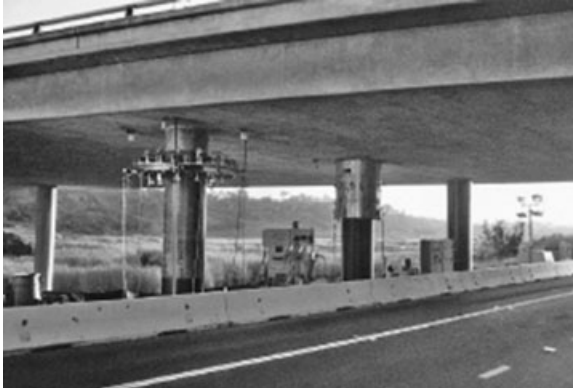
1.2 The XXsys carbon fibre jacket site filament winding technique (© XXsys Technologies Inc., San Diego, Ca, USA).
