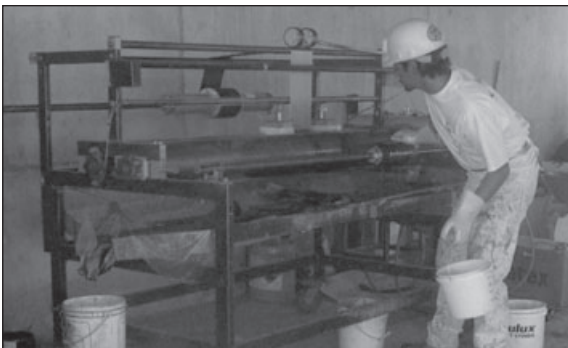
4.1 Impregnation of carbon fabric in wet lay-up process.
