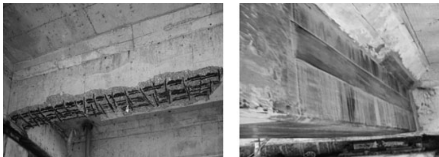
2.18 Scheifele Bridge – girder before and after repair.
