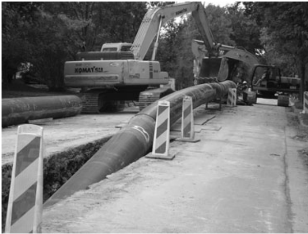
10.6 Typical continuous sliplining process.
