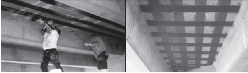
4.2 Application of wet lay-up CFRP composites to deck soffit.
