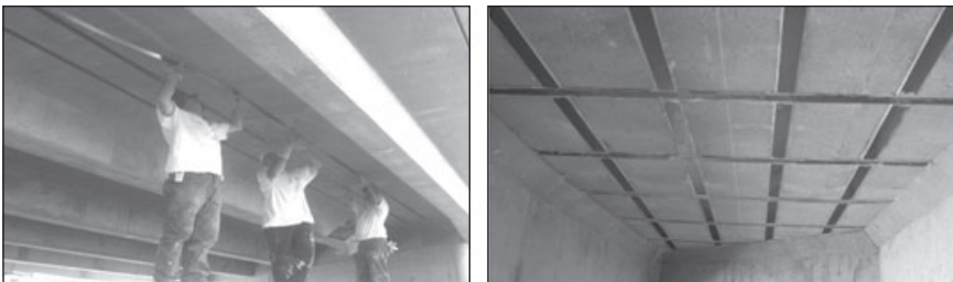
4.4 Bonding of pultruded CFRP strips to deck soffit.
