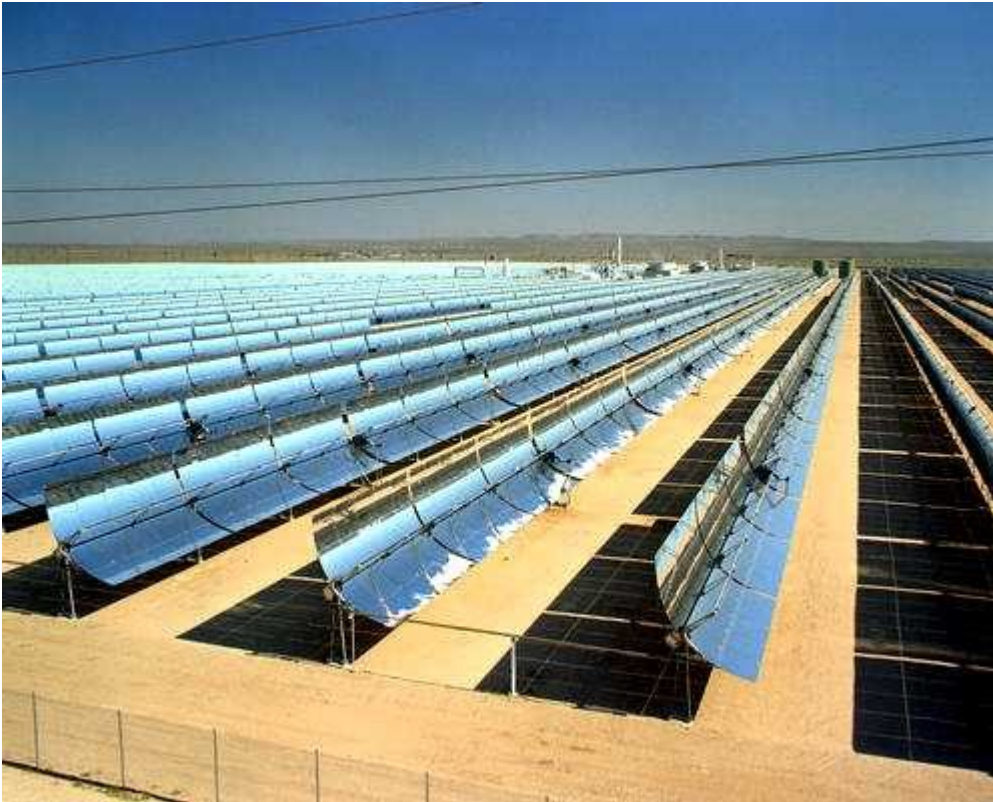
Figure 1.1 One of nine solar electric energy generating systems at Kramer Junction, California, with a total output of 354 MWe. (photo courtesy Kramer Junction Operating Company)
