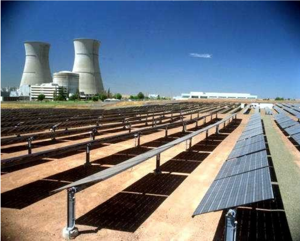
Figure 1.2 A 2-MW utility-scale photovoltaic power system co-located with a defunct nuclear power plant near Sacramento, California. (photo courtesy of DOE/NREL, Warren Gretz)
