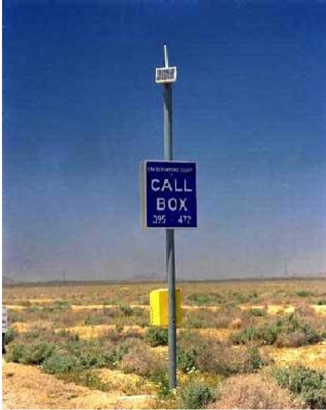
Figure 1.8 Flat-plate photovoltaic collector applications.(photos courtesy of DOE/NREL, Warren Gretz)
