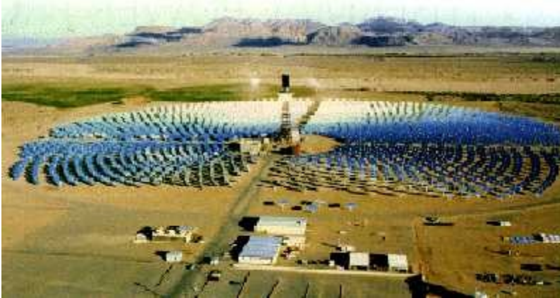
Figure 1.10a A central receiver system. (courtesy of Sandia National Laboratories, Albuquerque)
