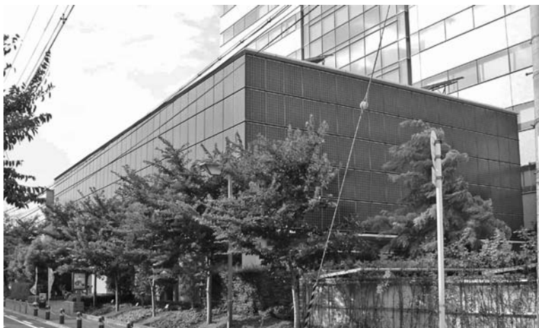
FIGURE 8.14 Sanyo corporate headquarters in Tokyo with BIPV on the south, east, and west sides of this office complex.
