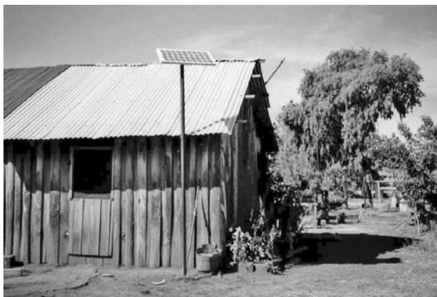
FIGURE 8.17 Solisto 50 W p PV lighting system installed in Talayotes, Moris County, Chihuahua.
