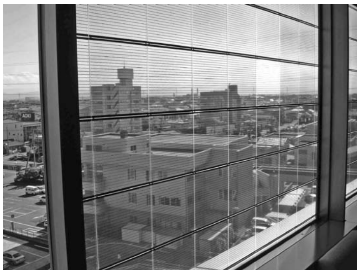
FIGURE 8.11 Building integrated see-through PV modules (Sanyo) at the Ohta City government office complex.
