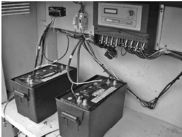
FIGURE 8.20 Battery charging at Francia Sirpi with Stecca controller capable of charging eight batteries simultaneously.
