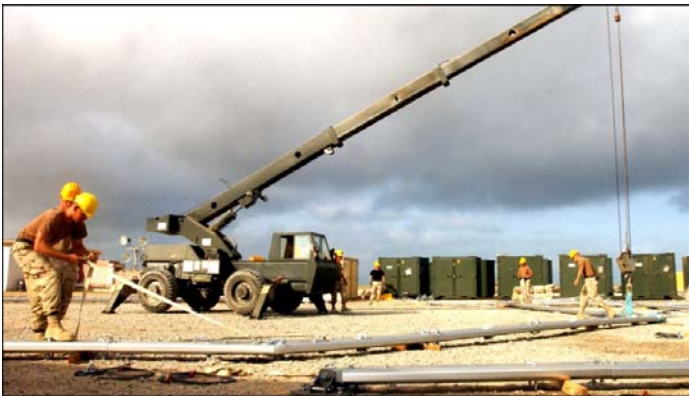
Figure 1.3. 49th MMG Assembles Large Area Maintenance Shelter.
