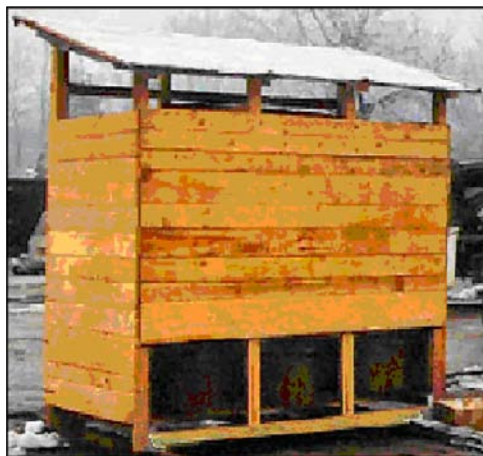
Figure 6.13. Portable Burn-Out Latrine.
