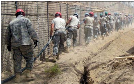
Figure 9.8. Burying Electrical Distribution Cable.
