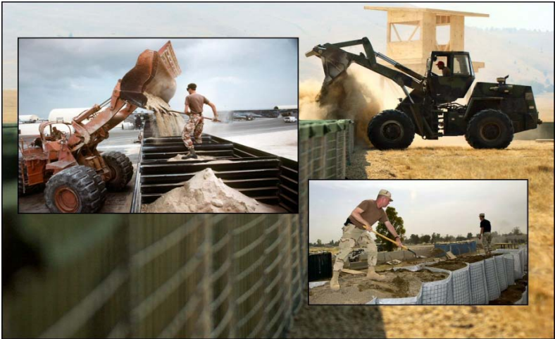
Figure 4.12. Expedient Revetments at Deployed Locations.
