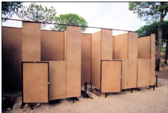
Figure 6.4. Straddle Trench Latrine with Partitions.
