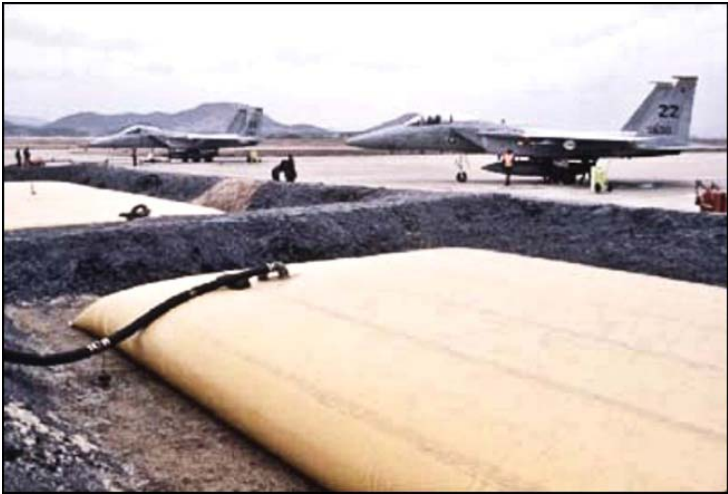
Figure 4.14. Fuel Dikes Around Jet Fuel Storage Bladders.
