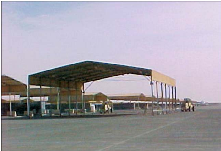
Figure 5.7. Engineers Relocate Aircraft Sunshades.
