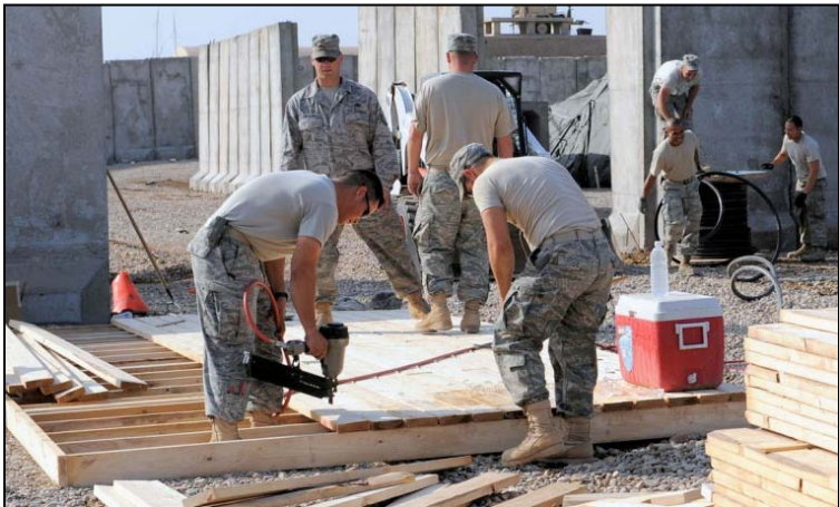
Figure 5.9. Building Army Shower Facilities at an FOB.
