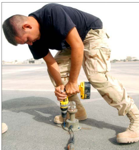
Figure 4.7. EALS Supports Contingency Airfield Lighting Requirements.
