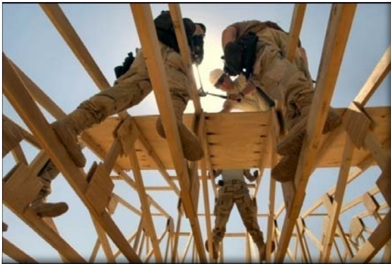
Figure 1.6. Building an Army TOC at FOB Kalsu, Iraq (2007).
