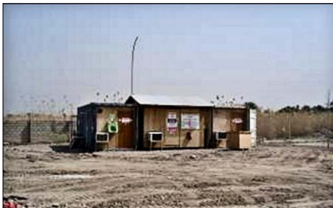
Figure 7.4. Isolated Pesticide Storage Facility at Deployed Location.
