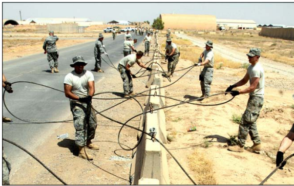
Figure 11.5. Constructing Security Barrier around Flightline.
