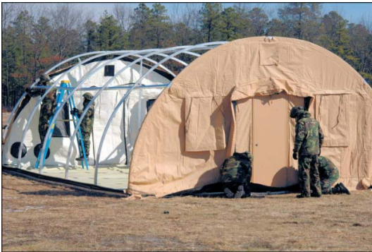
Figure 11.2. Erecting Non-Hardened BEAR Shelter.
