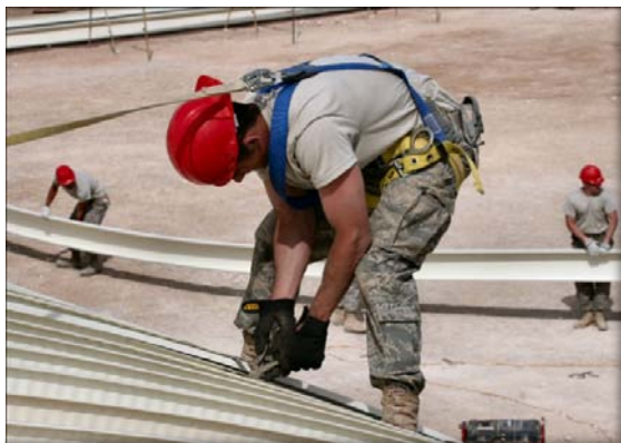
Figure 1.2. RED HORSE Constructing Warehouse Facility in Iraq (2008).
