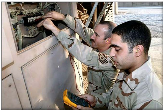
Figure 1.4. CEMIRT Members Perform Depot-Level Repairs.
