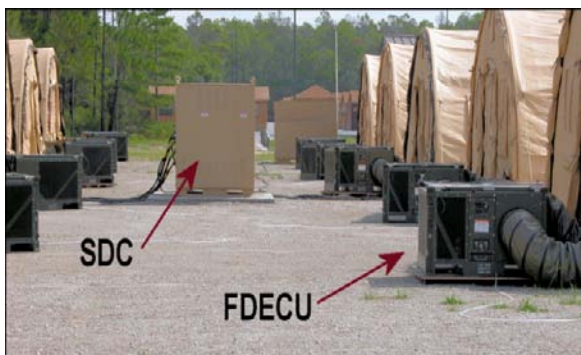
Figure 9.6. Typical SDC/Facility Configuration with FDECUs.
