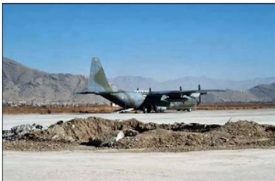
Figure 4.6. Crater with Upheaval.
