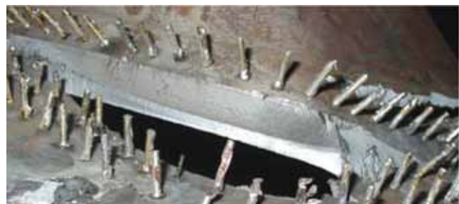
Figure 1. Crack surface of Y-joint specimen
