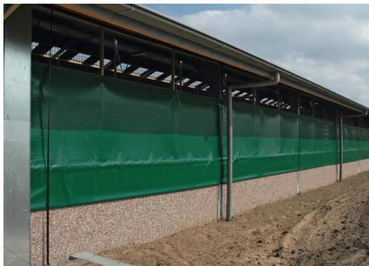
Our curtain system features maximum air flow with minimum air restriction. Temperature sensors allow control for complete automation. They can be manually or automatically operated based on each dairy's needs. All curtains are installed by trained technicians that will ensure
