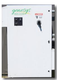
The Livestock Comfort System by Genesys Energy Systems is an all-in-one, automated barn ventilation management system that provides significant energy savings, paying for itself in as little as three years. The only system of its kind on the market, the Livestock Comfort System is a complete power and control system. A single system automatically controls and adjusts fan speed, curtains, alarms, lighting and sprinklers both inside and outside the freestall barn. Experience year-round benefits of
