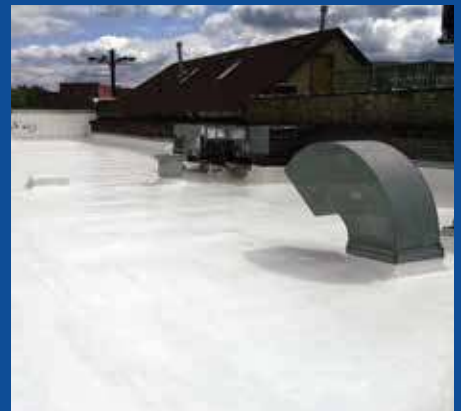
Liquid-Applied Roofing
