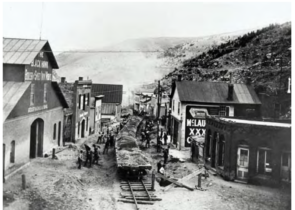
C & S temporary track in Main Street of Black Hawk after the 1910 flood.
