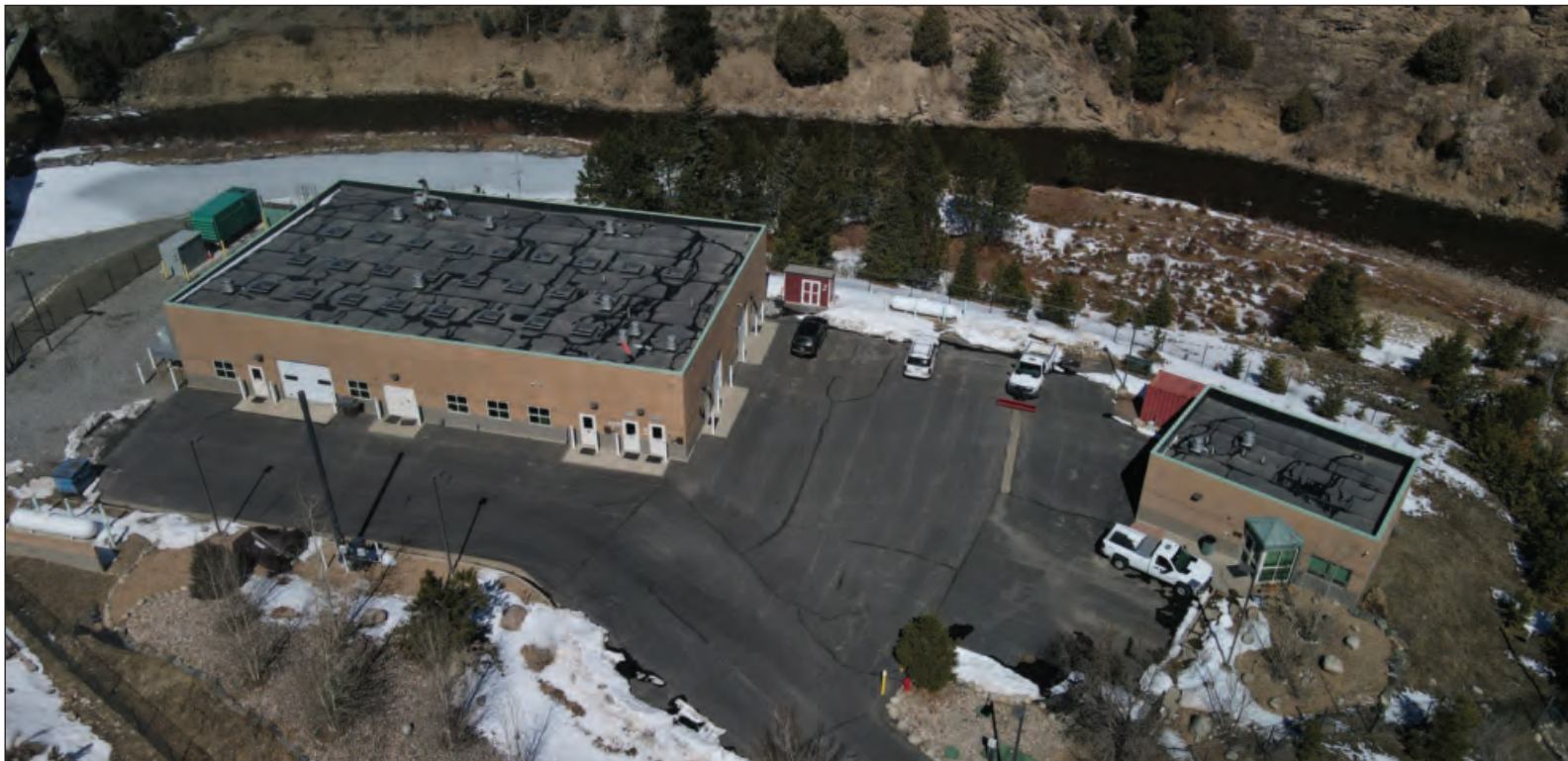
Black Hawk’s water treatment plant, near the Central City Parkway at I-70, draws water from Clear Creek. The water is treated and piped uphill for seven miles to a storage tank at Miner’s Mesa.
