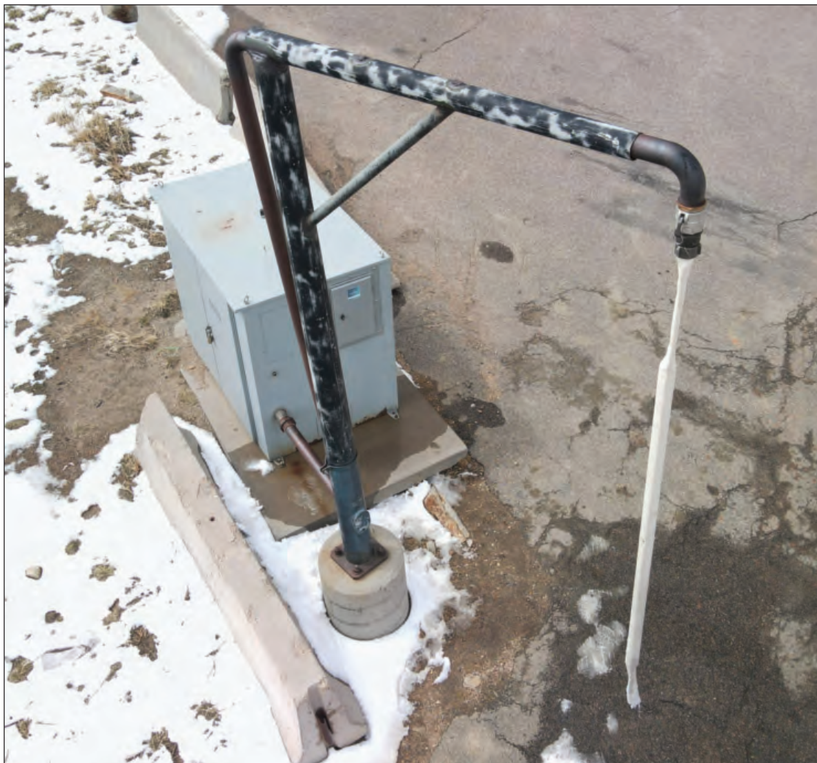
Central City sells its municipal water to Gilpin County residents via a bulk water-dispensing machine near the KOA campground. Registered users swipe a credit card on the unit and fill containers they bring with the same water the city delivers to homes, businesses and casinos.
